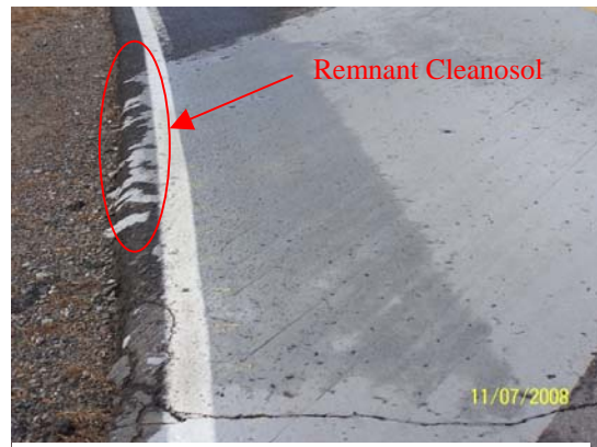
Brown Road, Groveton Edge Wear of Cleanosol (End Strip is Worn Away Due to Lack of Shoulder Material)
