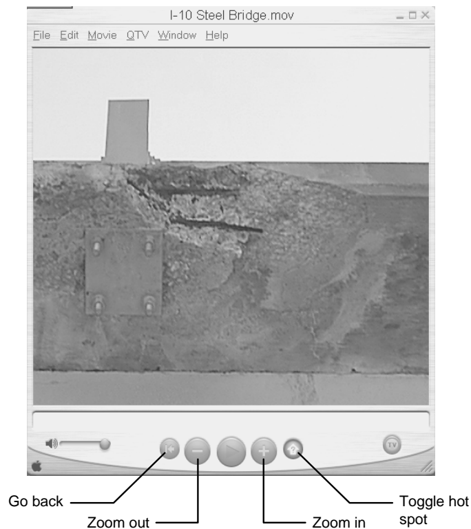
FIGURE 5 Virtual Reality Record of Reinforced Concrete Deck Showing Display Buttons.
