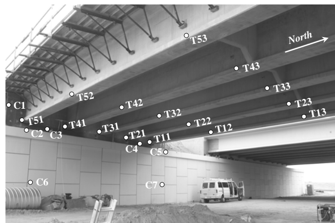
Figure 5. Locations of tie and control points on Las Alturas Bridge.
