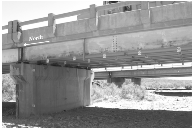
Figure 8. Target layout towards north end of Alamosa Canyon Bridge.
