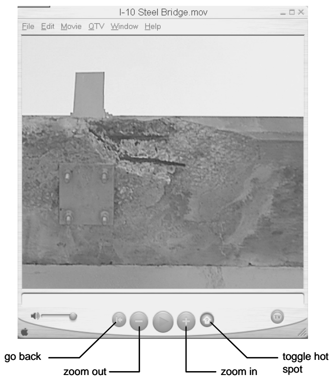
Figure 4. Virtual reality record of reinforced concrete deck showing display buttons.
