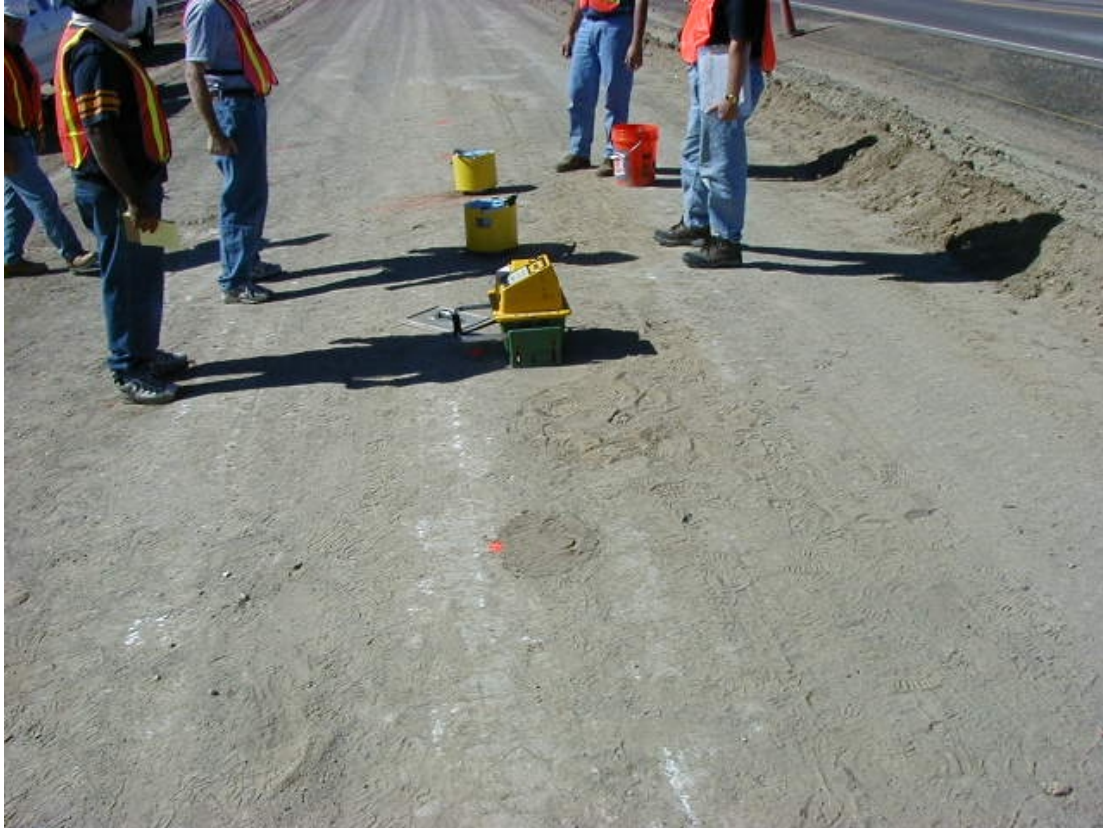
Figure 27. Field Measurements on Lime Stabilized Subgrade.
