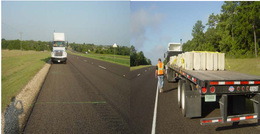
Figure 25. Loaded Test Truck along the Test Segment.
