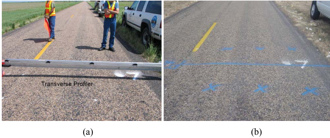
Figure B10. FM 28 Location 2 on Milepost 182+2100' (a) July 11th; (b) December 6th.
