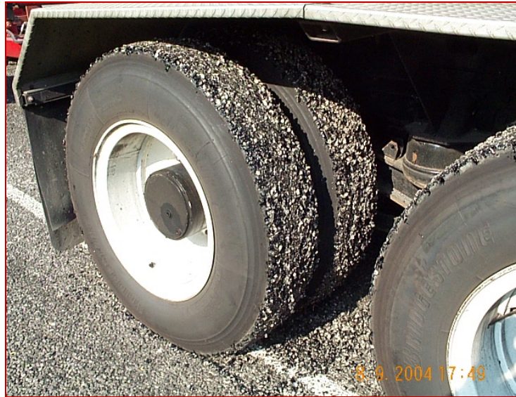
Figure 1. Seal Coat Damage due to SHL Moves.
