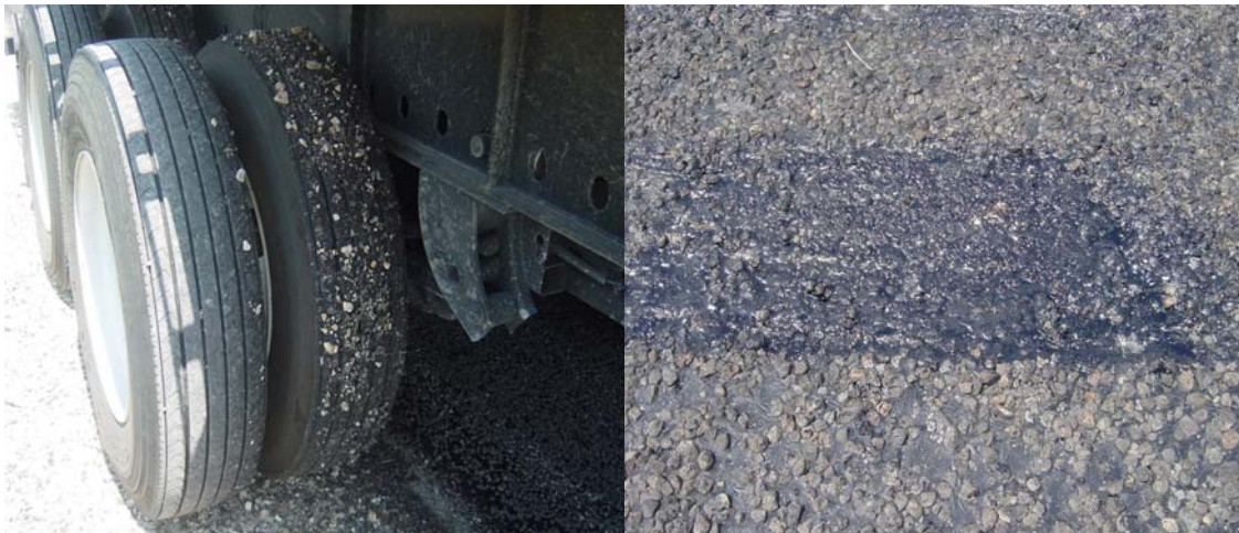
Figure 29. High Level of Damage.
