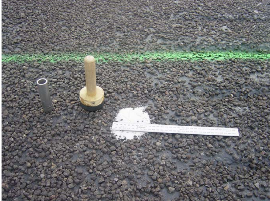
Figure 32. Sand Patch Test Conducted.
