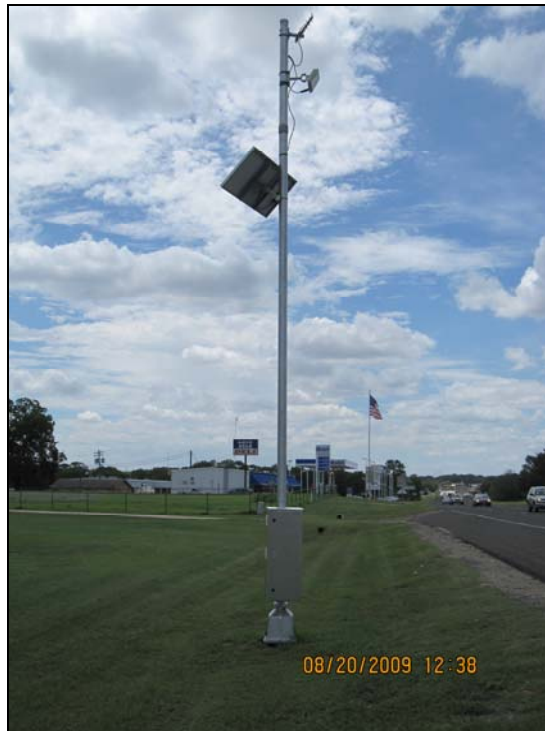
Figure 5. Reinstalled Equipment at the Caldwell Site.
