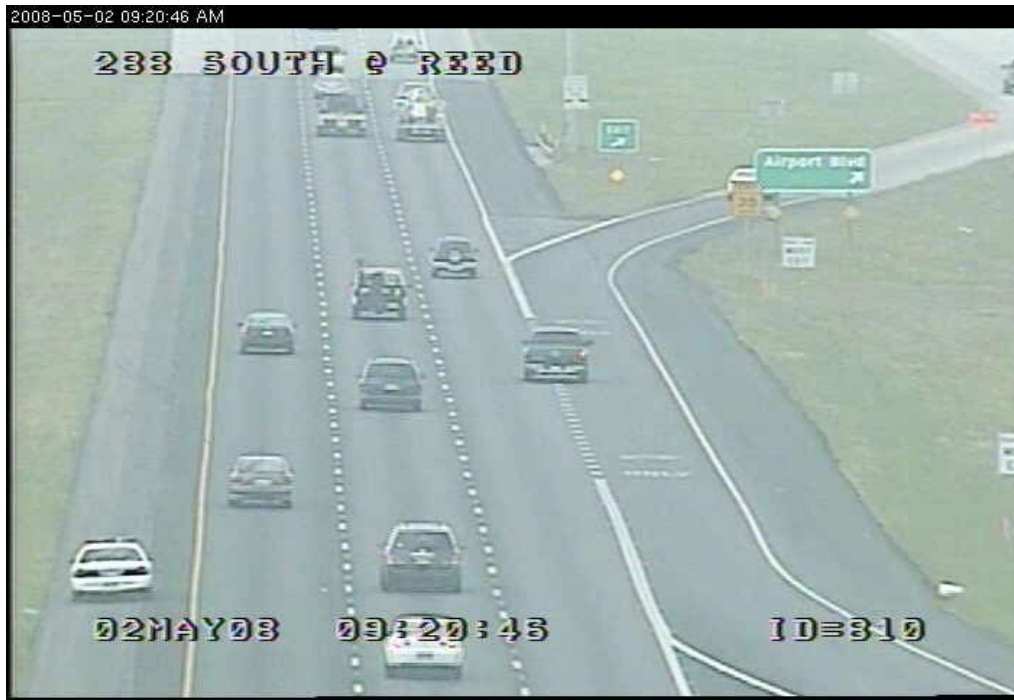
Figure 3-1. View of SH 288 SB between Reed Road and Airport Boulevard (Viewed from Camera 810 at Reed Road).
