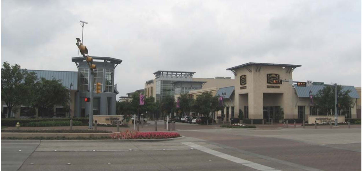
Figure A-2. Legacy Town Center Retail, Restaurant, Cinema Buildings along Retail Main Street.
