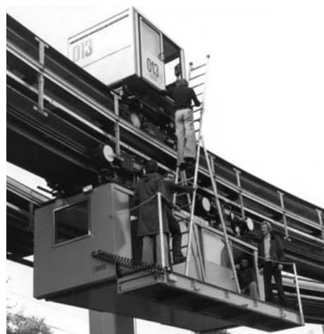
Figure 18 - Cabintaxi Emergency Evacuation
