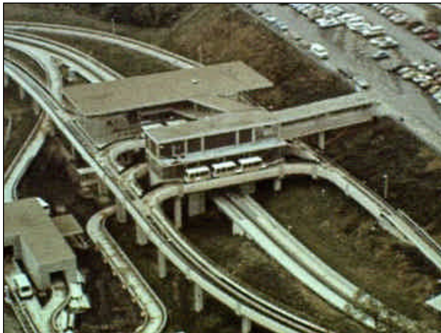
Figure 3. Engineering Station: 6 channels, bypass underneath the station, and adjacent maintenance facility. Photo from http://faculty.washington.edu/~jbs/itrans/morg.htm .
