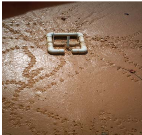
Figure 18. Faircloth Skimmer submerged and clogged with sediment.
