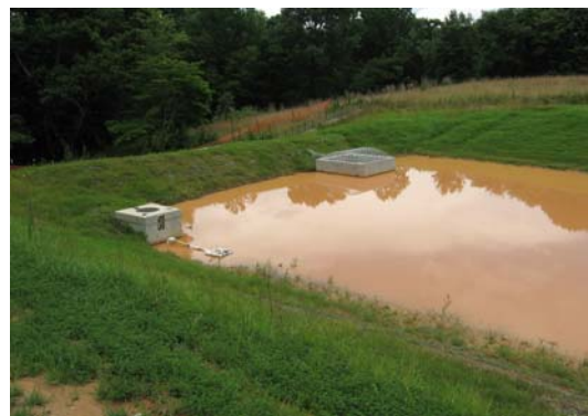
Figure 14. Proper installation of 2:1 sloping walls with ground vegetation established.
