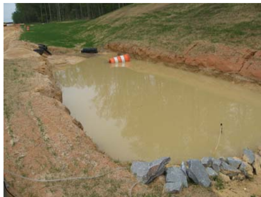
Figure 8. Standard Trap with standing pool 2 (STSP2 ) with vertical walls
