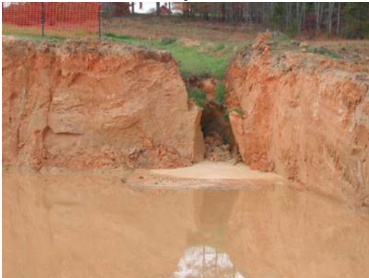
Figure 11. An estimated four tons of soil eroded from the corner gully
