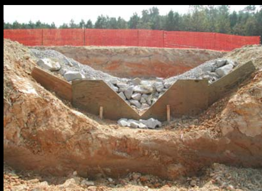
Figure 6. Standard Trap (10ST) with a V-notch weir installed to monitor and calculate flow.
