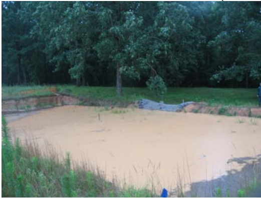
Figure 9. Standard 25-year Trap (25ST) during a substantial rainfall.
