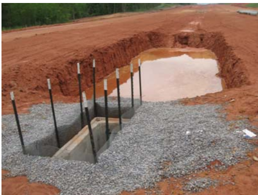
Figure 7. Standard Trap with standing pool 1 (STSP1) with vertical walls
