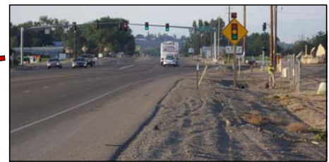
Traffic signal has good visibility from both directions
