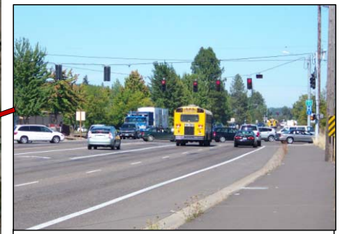
Traffic signal has good visibility
