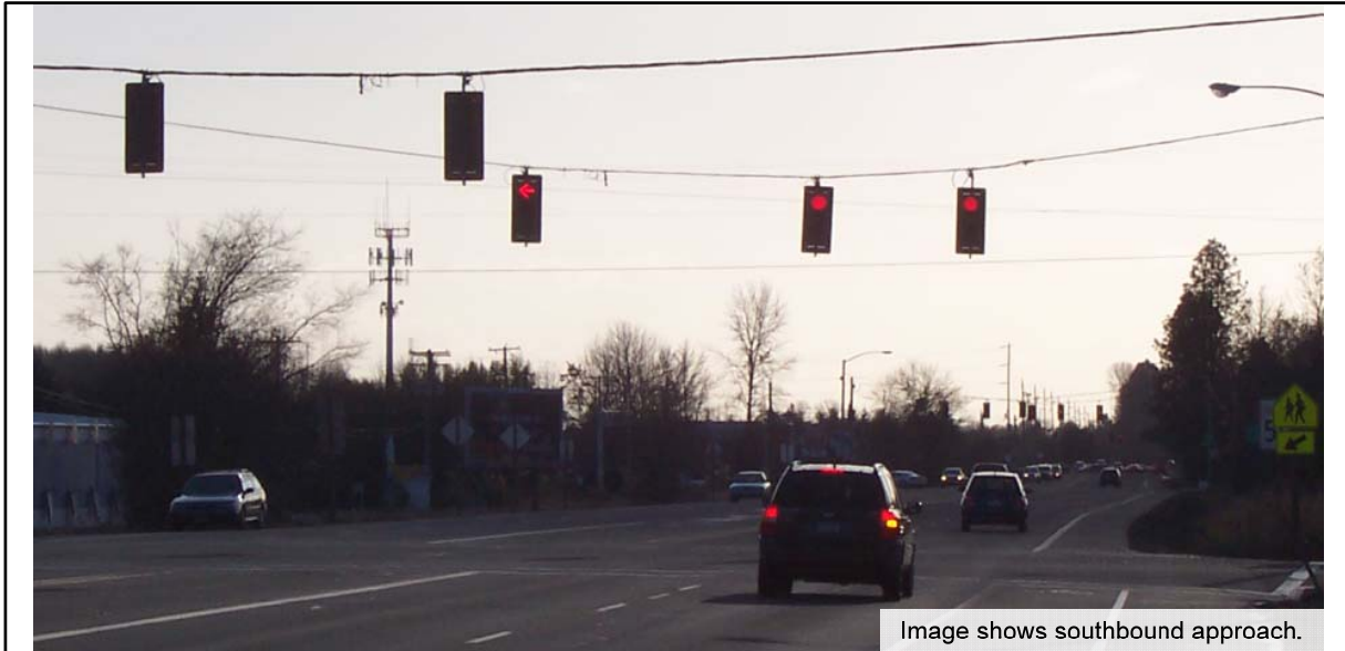
Picture showing typical arrangement and number of signal heads
