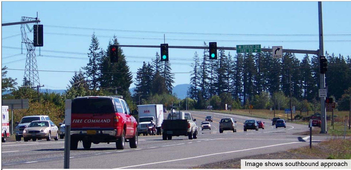
Picture showing typical arrangement and number of signal heads
