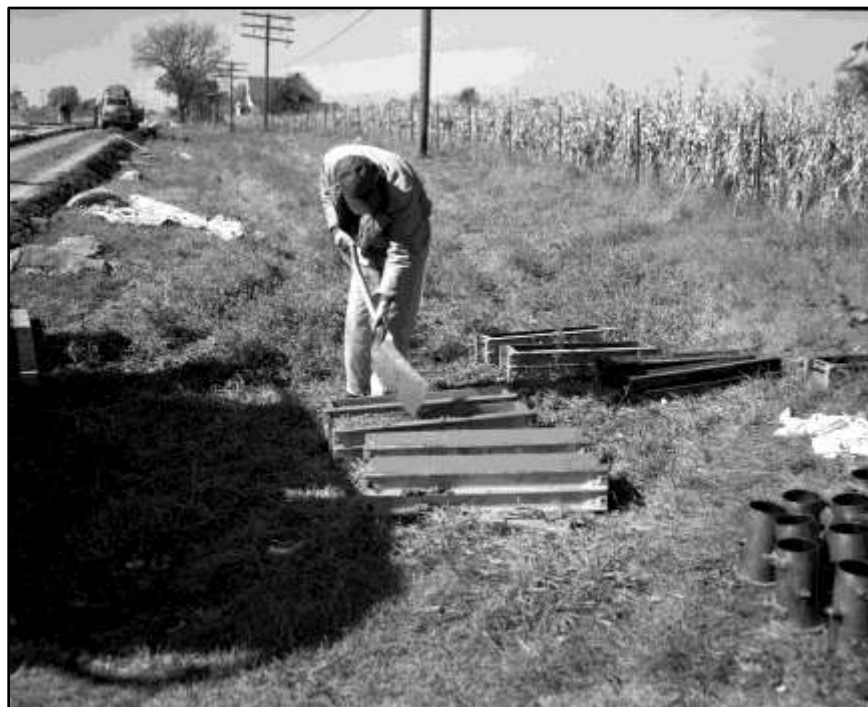
Figure 50 – Worker casting flexural strength specimens
