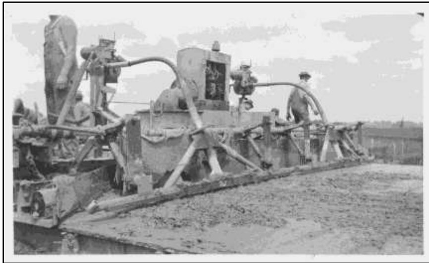
Figure 37 - Vibrators and tubes – Fayette County 1936
