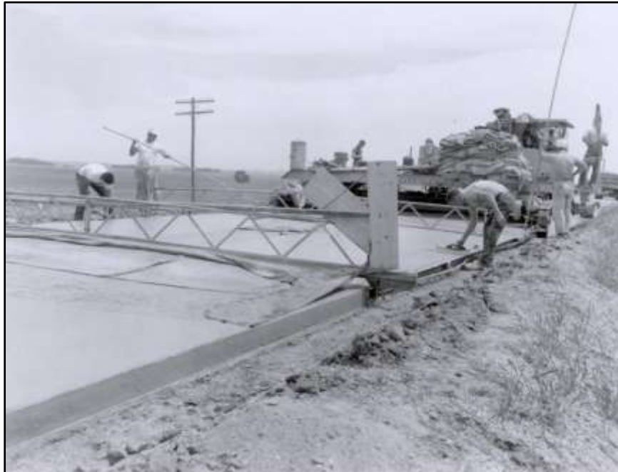
Figure 31 - Quad City slip form paver – Palo Alto County 1957
