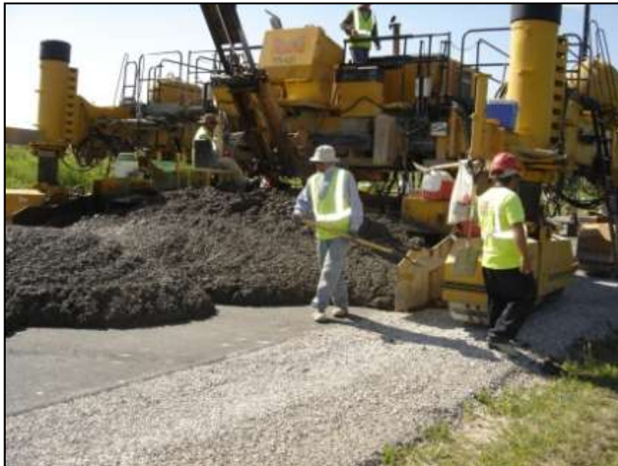
Figure 77 – String less paving – Poweshiek County 2009
