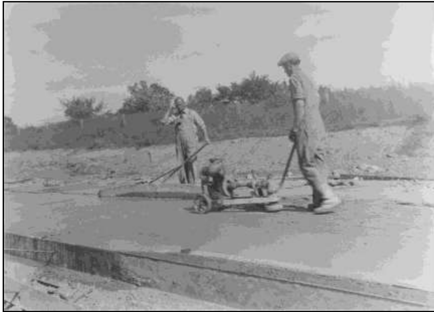
Figure 63 - Surface correction with carborundum brick – Keokuk County 1932
