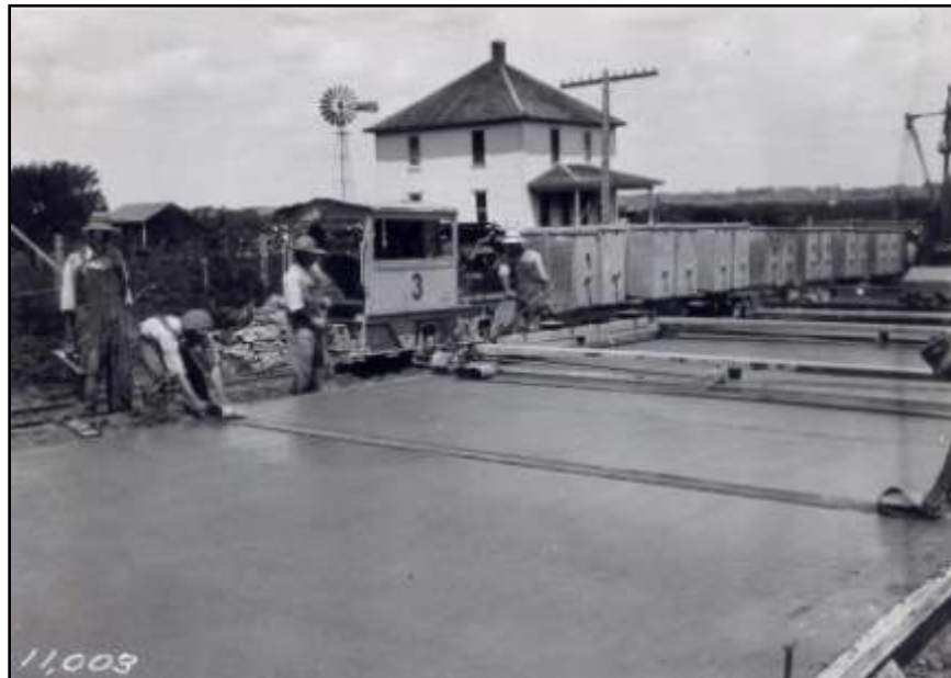
Figure 41 - Belting surface – Polk County 1926
