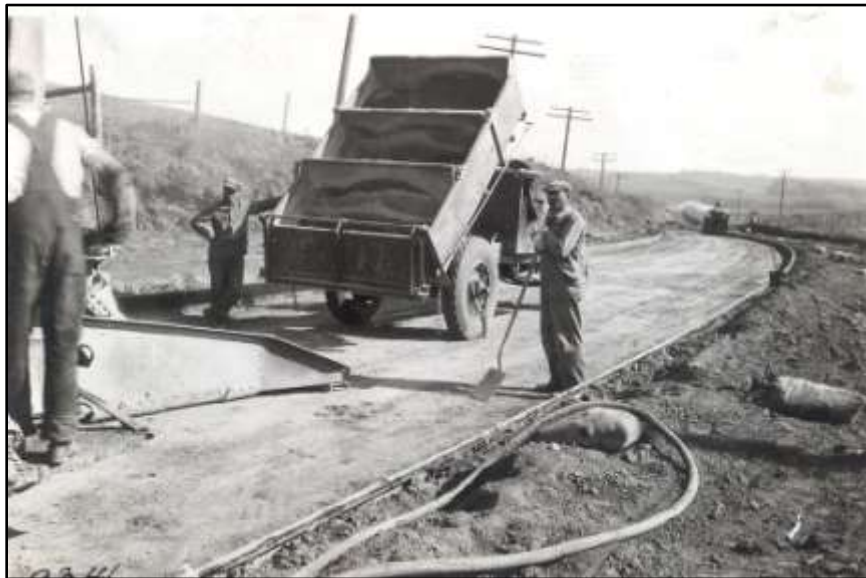
Figure 17 - Truck dumping into skip hoist - Woodbury 1921
