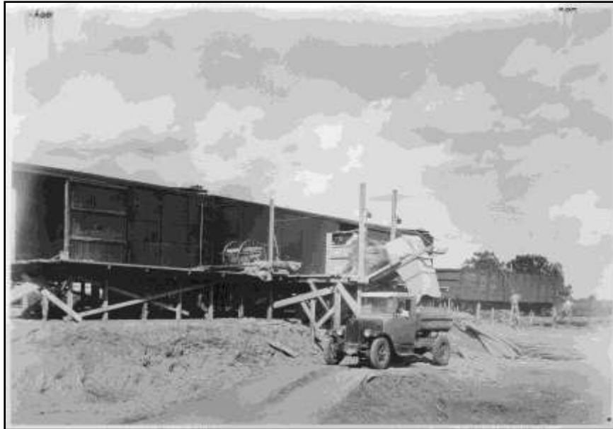
Figure 18 - Bulk cement dumping into truck – Howard County 1931
