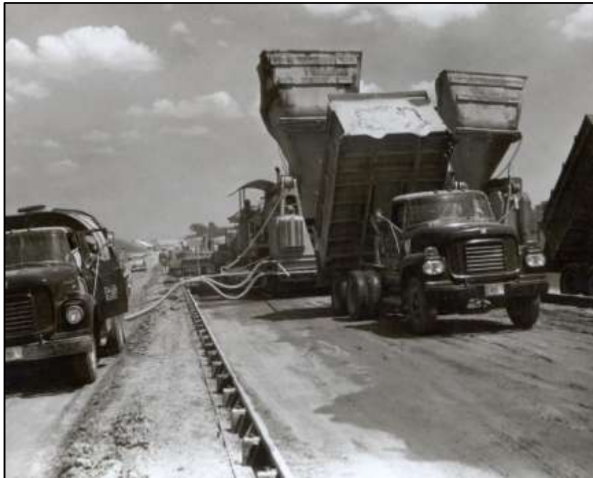
Figure 22 - Twin 34E mixers - Story County U.S. 30 1964
