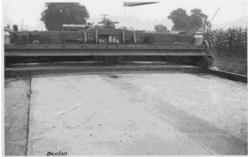
Figure 75 - PCC widening and resurfacing U.S. 30 Benton County 1949
