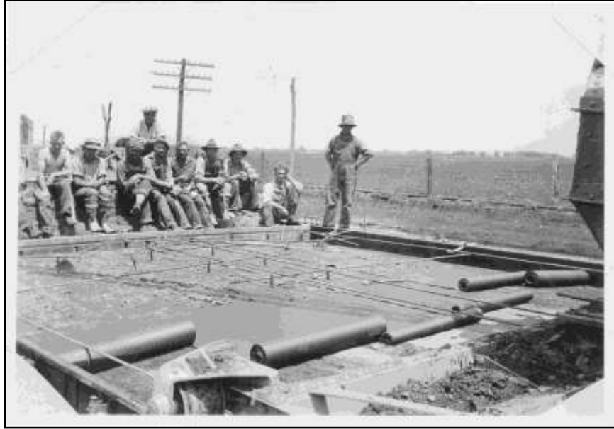
Figure 5 - Placing tar paper on subgrade - Story County 1926
