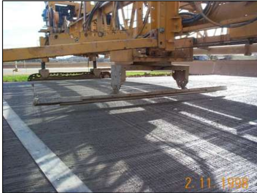
Figure 42 - Transverse tining - 1998
