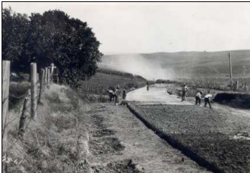
Figure 45 - Earth curing - Woodbury County 1921
