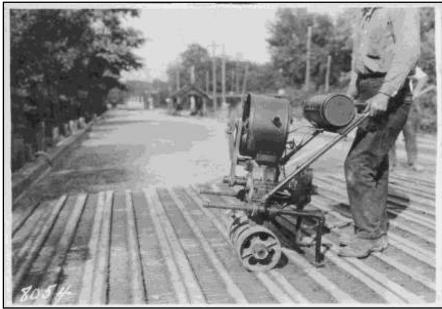
Figure 28 - Mechanical tamping and boards – Blackhawk County 1921
