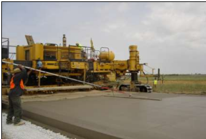
Figure 34 – Gomaco slip form paver - Henry County 2005
