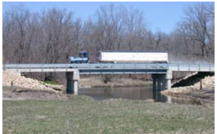
Figure 29 - The center span of the bridge uses pi girders (three individual units tied together) on a 50-foot span.
