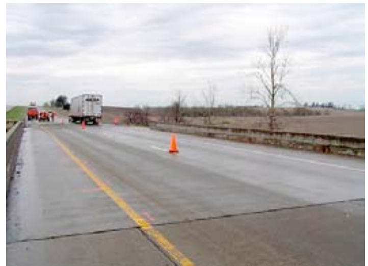
Figure 9 - Slab bridge on I-80 near Grinnell
