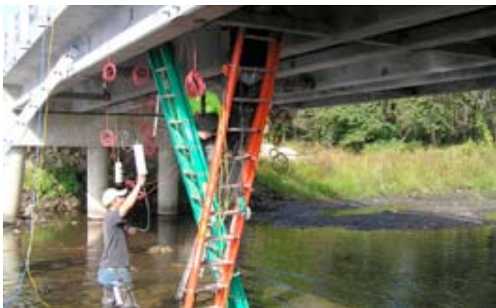
Figure 32 - Strain instrumentation placed on the pi-girder bridge prior to load testing.
