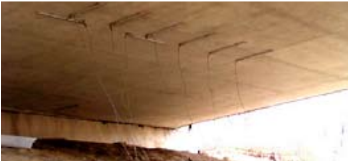
Figure 11 - Strain gauges attached to bottom of slab, midspan of end span
