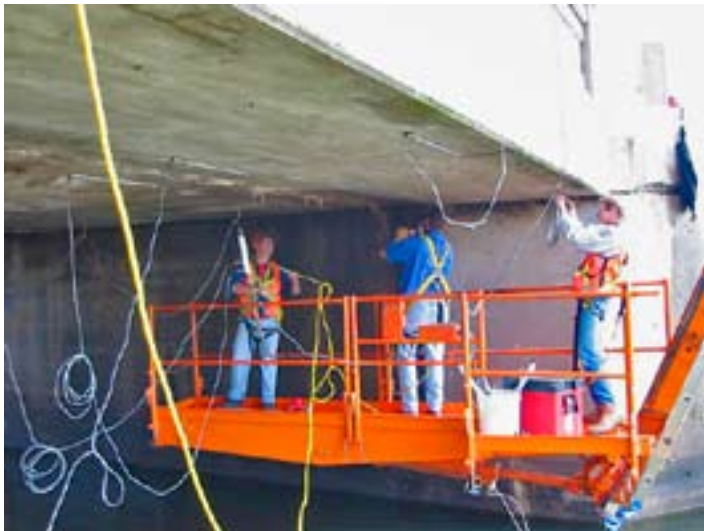
Figure 41 - Several BEC staff members placing instrumentation on a bridge
