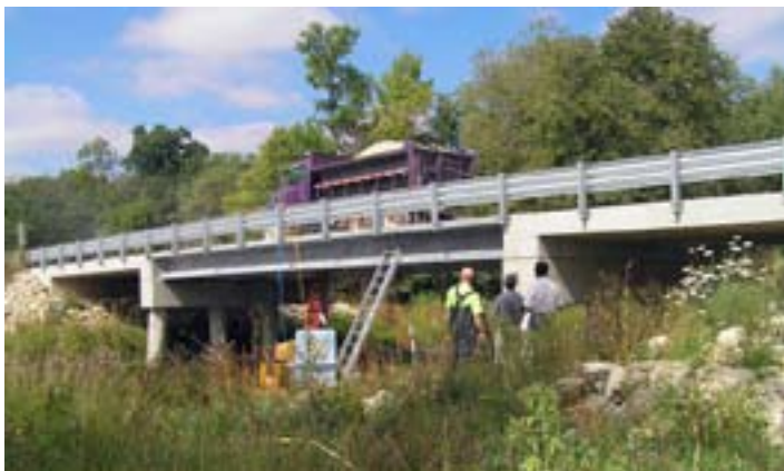
Figure 31 - Single-load test truck used for static and dynamic diagnostic load tests.
