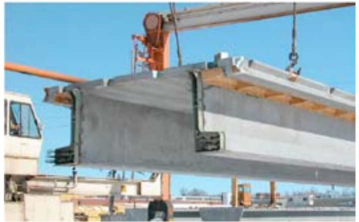
Figure 28 - New generation pi-shaped bridge girders utilizing UHPC.
