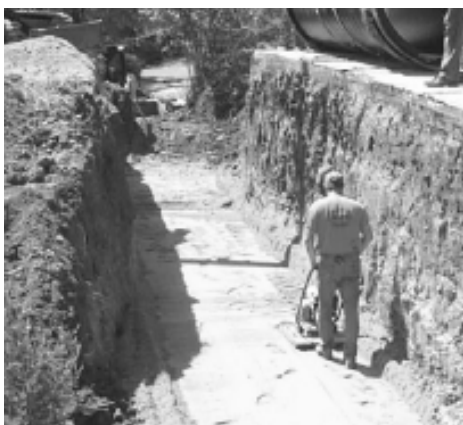
Figure 3. Pipe 2 Bedding Compaction
