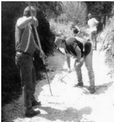
Figure 2. Pipe 1 Bedding Compaction
