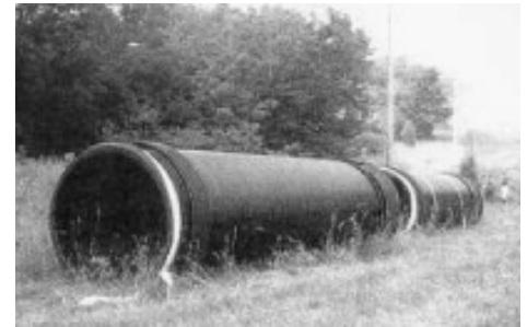
Figure 1 60" (1500mm) N-12 HC® HDPE Pipe
