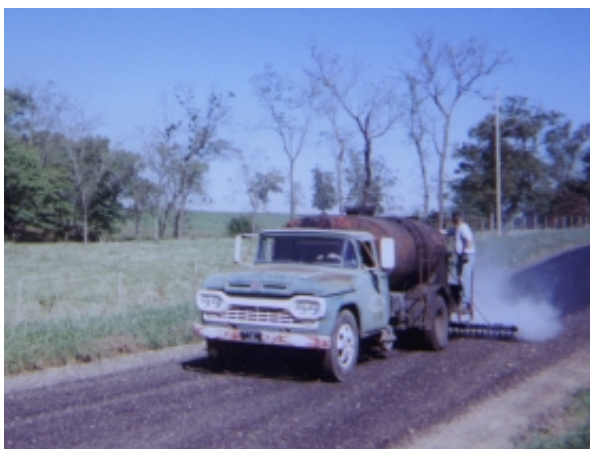
Tack is applied to the roadway. Oil is then added to the millings, mixed, placed and rolled.
