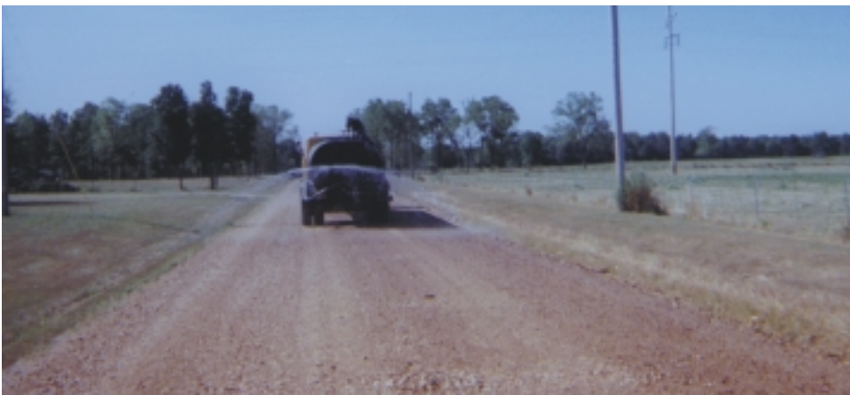
Roadway and ditches are reshaped, waste material is hauled off, roadbed is watered and compacted.
