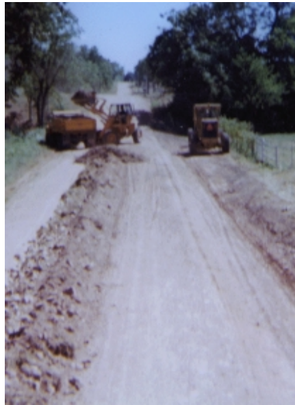
Roadway and ditches are reshaped, waste material is hauled off, roadbed is watered and compacted.
