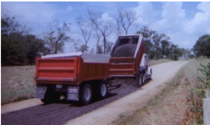
RAP millings are dumped, material is graded into wind rows for uniform thickness.
