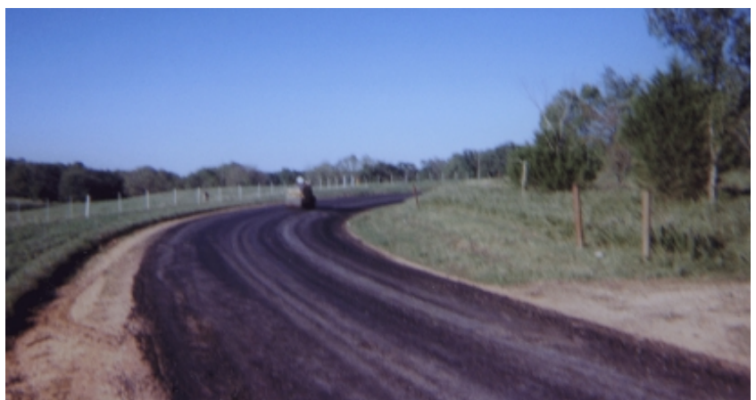
Tack is applied to the roadway. Oil is then added to the millings, mixed, placed and rolled.
