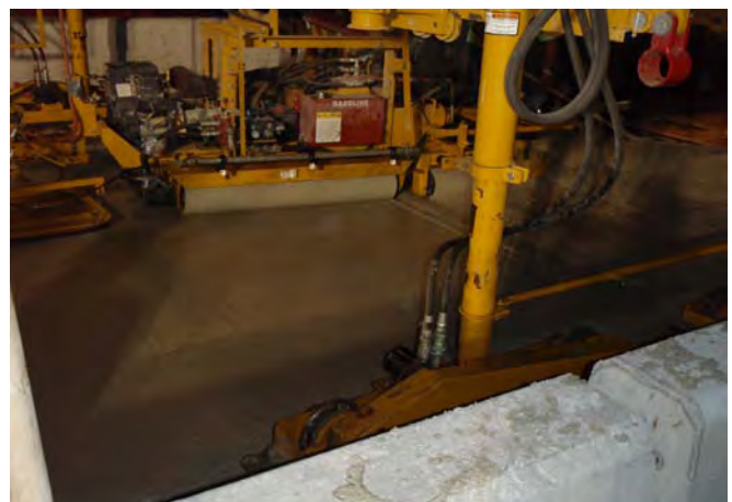
Bidwell bridge deck finisher.
