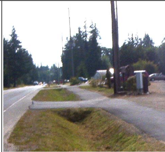
Figure E.5b: Crescent School after the SRTS project
