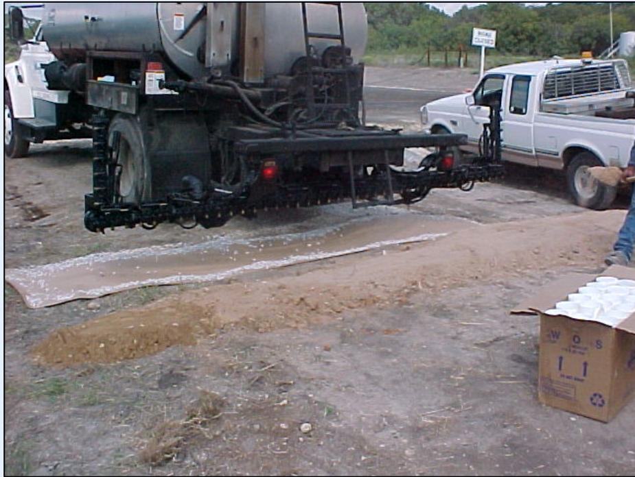
Figure 2 – Building Calibration Test Pad
