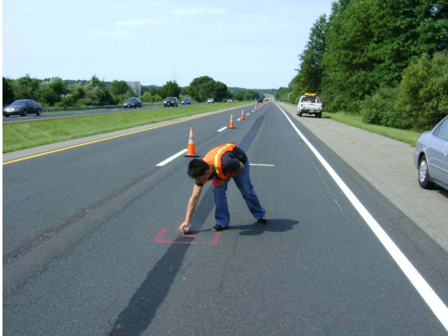
Figure 28: Site Preparations for Field Test Location of the Skid Test
