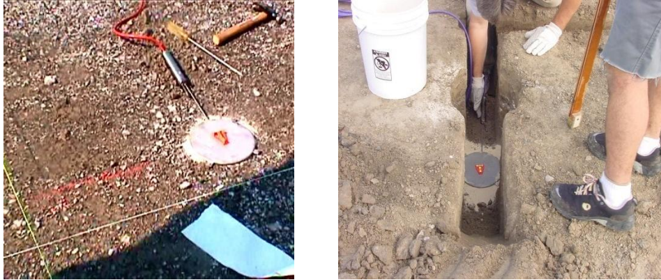
Figure 5 Installation of pressure cells at the ALF facility
