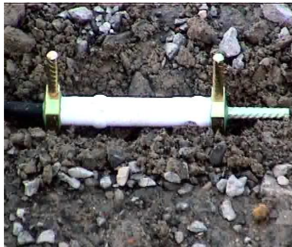
Figure 6 Installation of the strain gages at the ALF facility (Experiment III)
