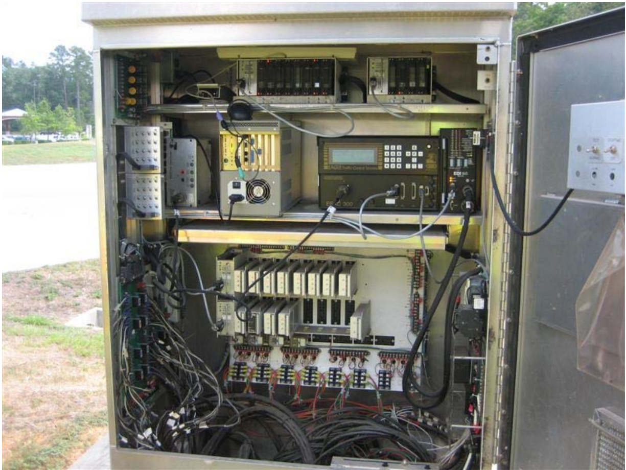
Figure 26. Installation of Adaptive D-CS in the Houston District near Conroe.
