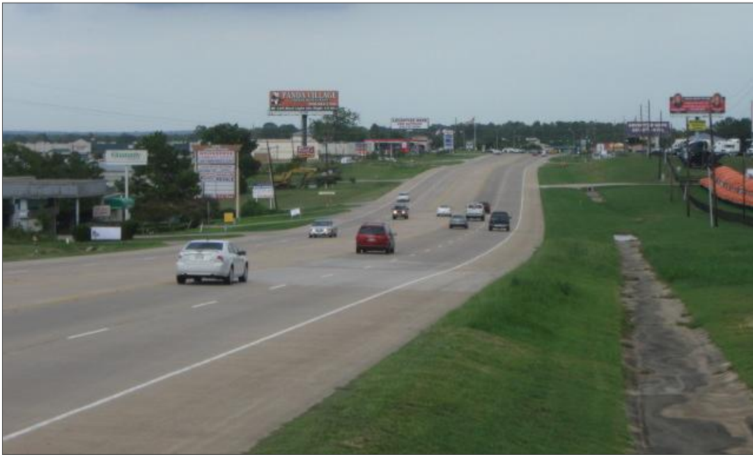
Figure 41. Existing 5-Lane Section of SH 105 on West Side of Corridor Study Area.
