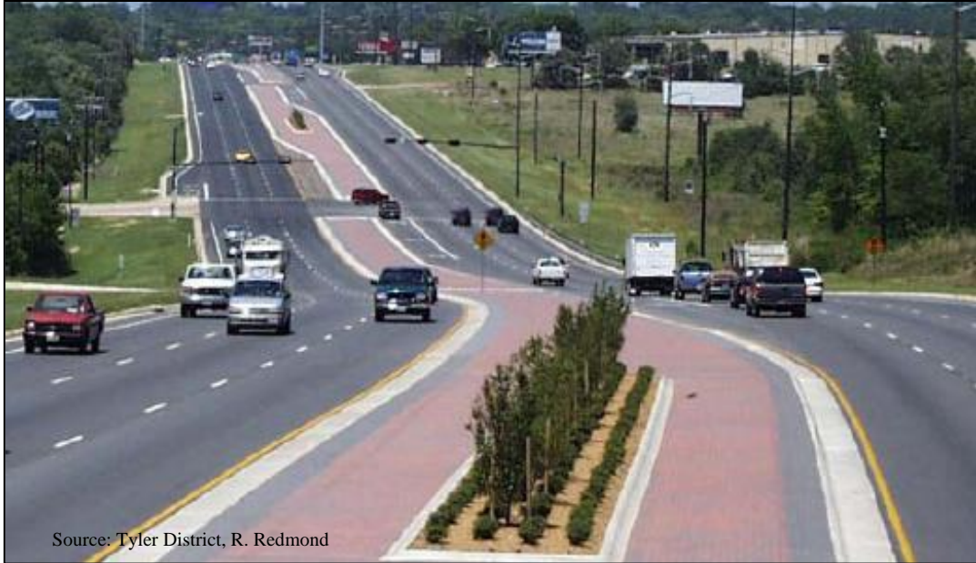
Figure 50. Loop 323 in Tyler: Example of High Speed, Multi-lane Arterial with Raised Median.
