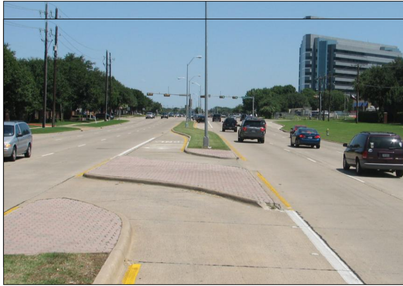
Figure 57. Hooded Left-Turn Design on Preston Road.
