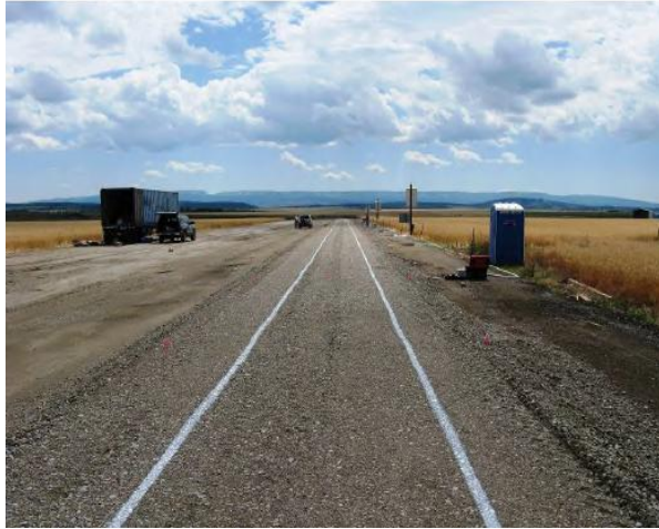
Figure 2.5: Full-scale field testing (Cuelho and Perkins 2009).
