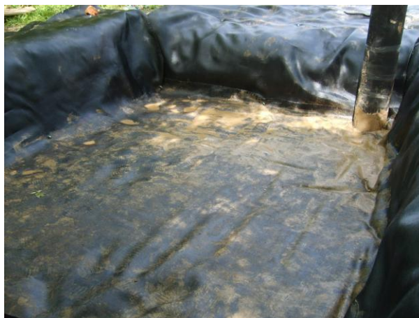
Figure 3.8: Geotextile lined test pit.
