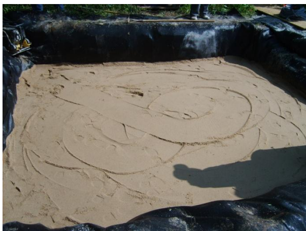
Figure 3.11: Compacted sand layer.
