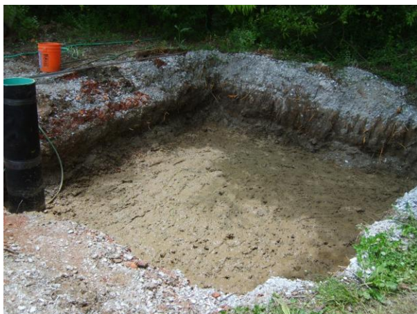
Figure 3.7: Construction of the test pit.
