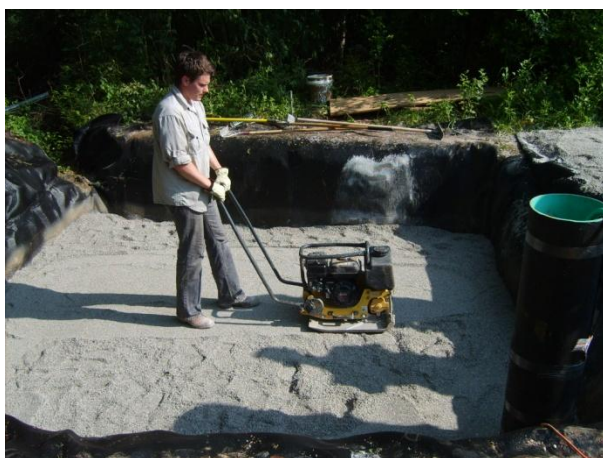
Figure 3.9: Compaction of 8'' gravel layer.
