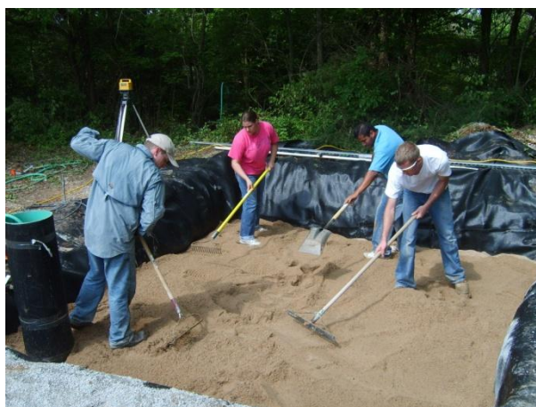
Figure 3.10: Placement of 6'' sand layer.
