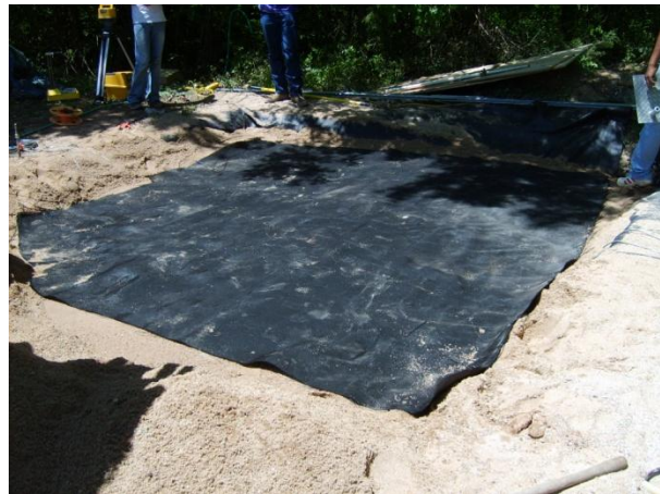
Figure 3.18: Geotextile placement.
