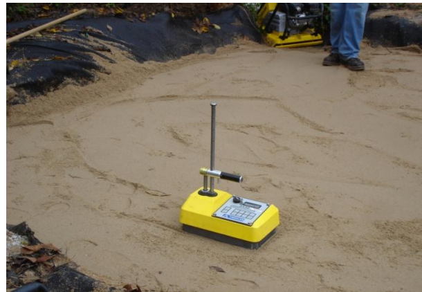
Figure 4.4: Nuclear density reading on the sand layer.
