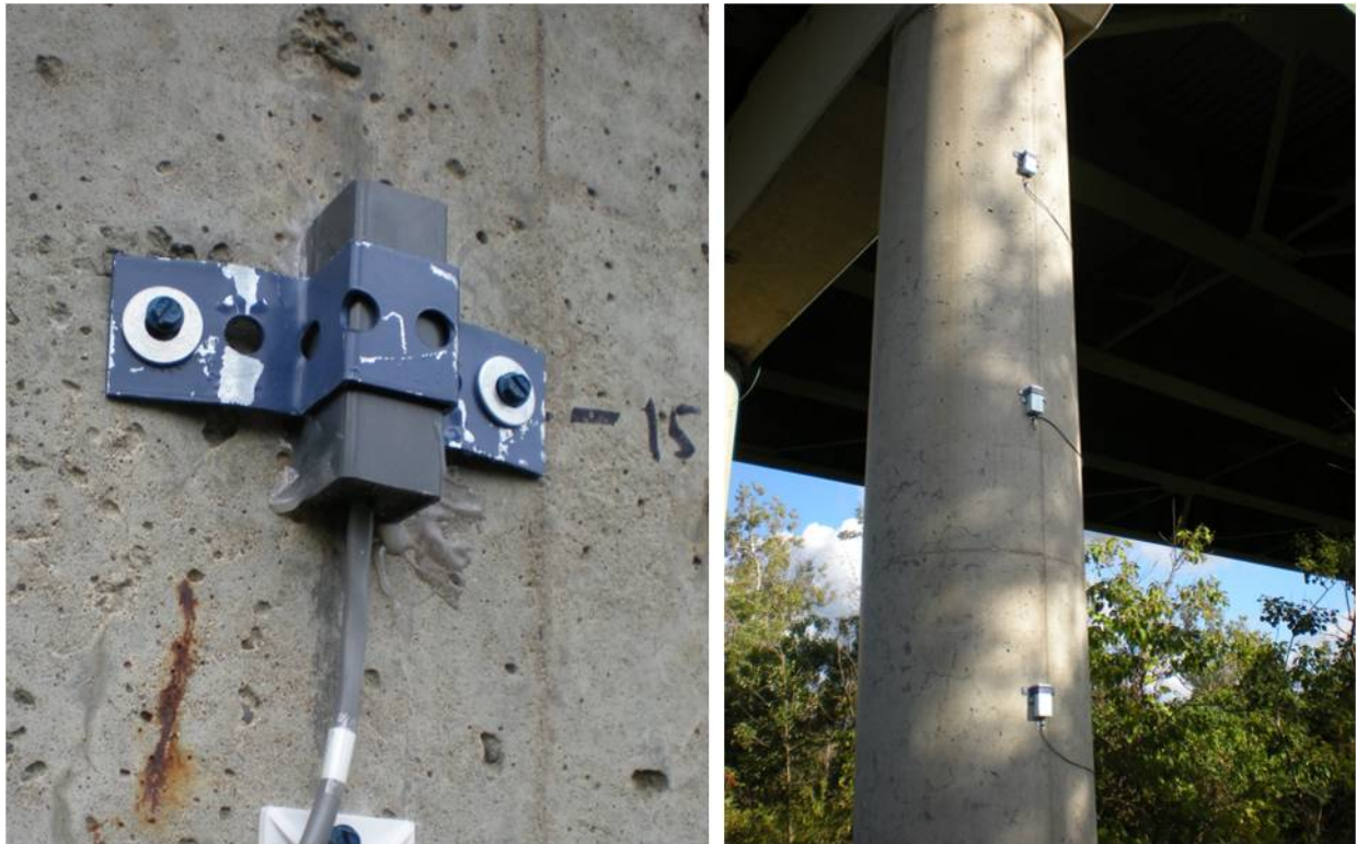
Figure 25. Sensors mounted on bridge: individual sensor (left) and a three sensor array (right).
