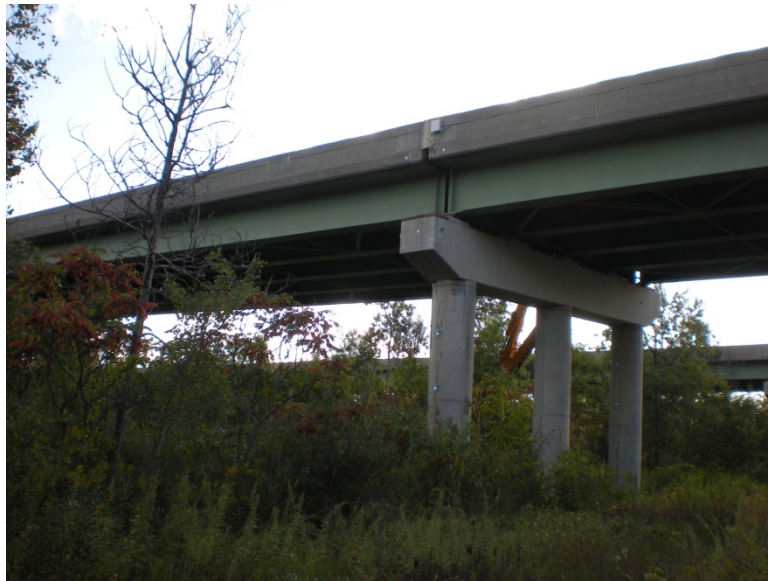
Figure 22. Photograph of pier three of the bridge.
