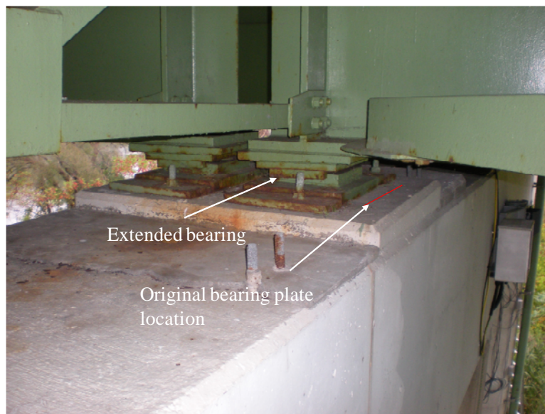
Figure 23. Photograph of expansion device at pier 3.
