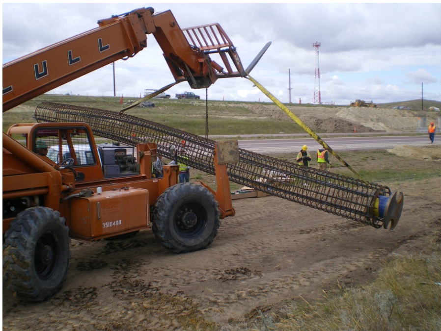
Figure 10. Test shaft reinforcing cage with attached O-cell (Photo by S. Cooney)
