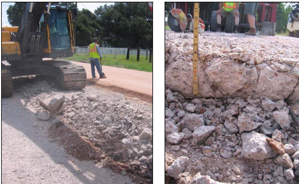
Figure 4.1. Rubblized Product from Type I (Left) and Type II (Right) Equipment.
