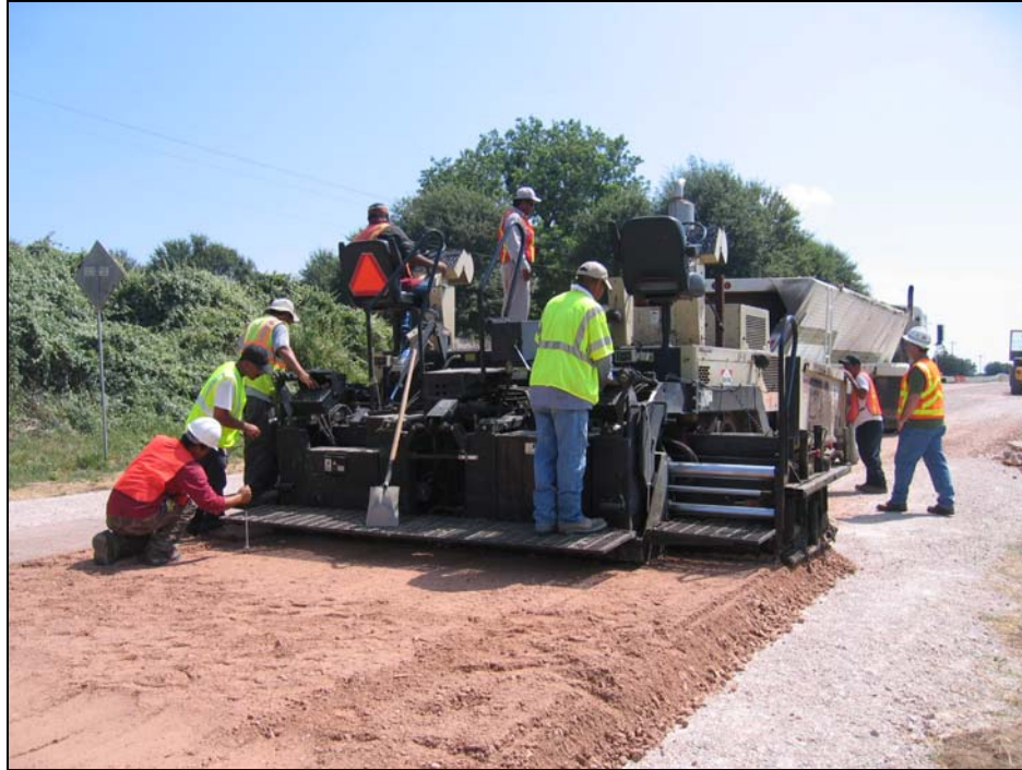
Figure 2.12. Placing Base with Paver.
