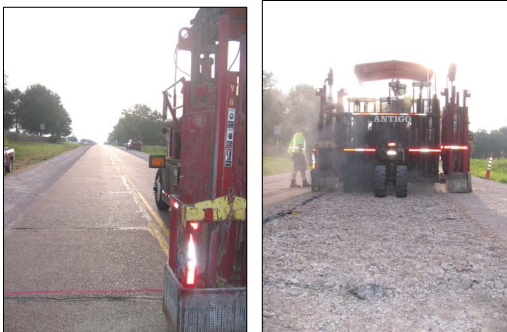
Figure 2.1. Unfractured (Left) and Rubblized (Right) JCP during Type II Rubblization.
