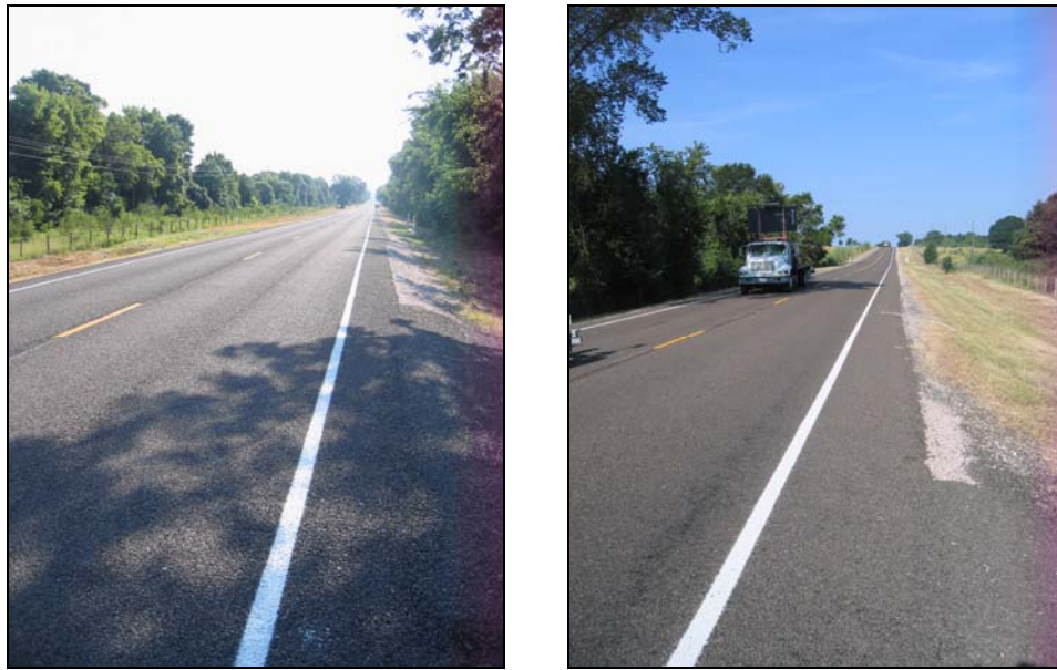
Figure 3.1. Existing JCP with Grade 4 (Left) and Grade 2 (Right) Overlay.
