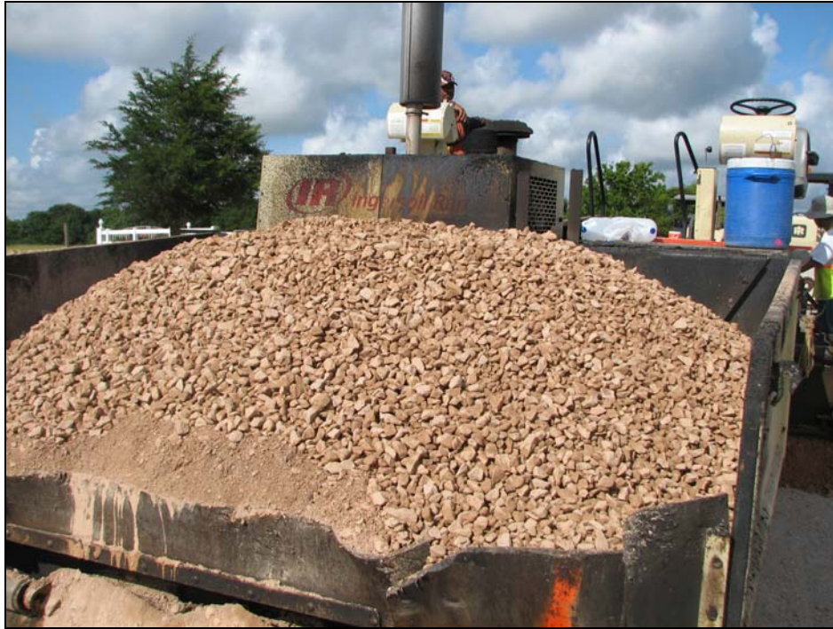
Figure 2.14. Segregation of Grade 4 Base in Paver Hopper.
