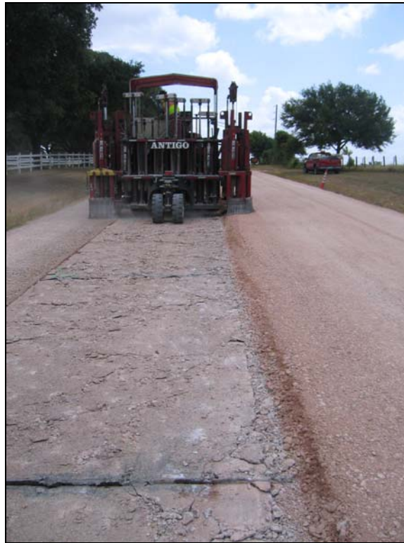
Figure 2.5. Modified Break Pattern with Type II Rubblization.
