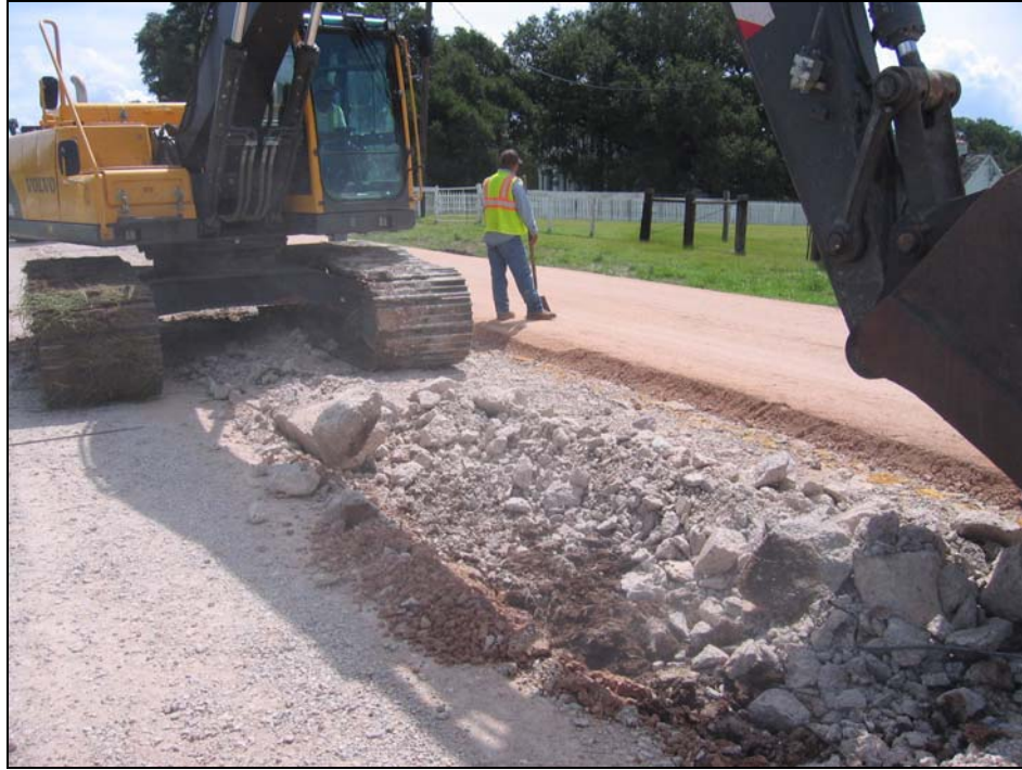
Figure 2.8. Test Pit with Type I Equipment.
