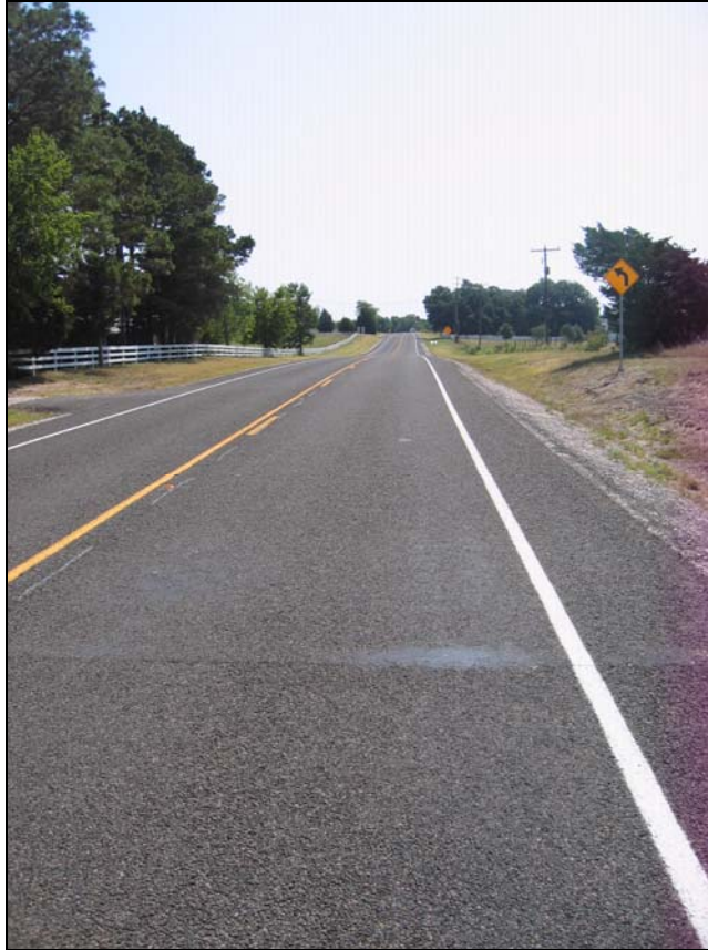
Figure 3.6. Start of Type I Rubblization with Grade 2 Base Overlay.
