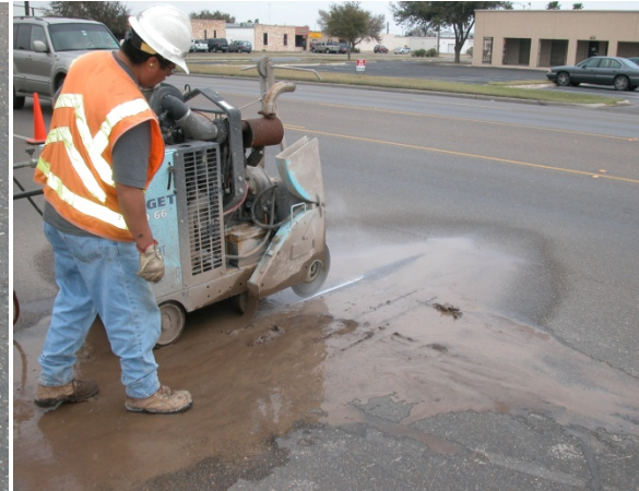
(b) Sawing Along the Template Marking
