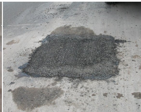
(f) Trench Filled up with Coldmix
