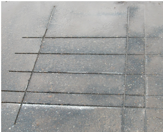
(c) Pavement after Saw Cut
