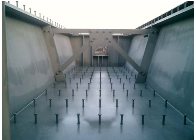
Figure 2.6 Shear Connectors and Interior Cross Frames
