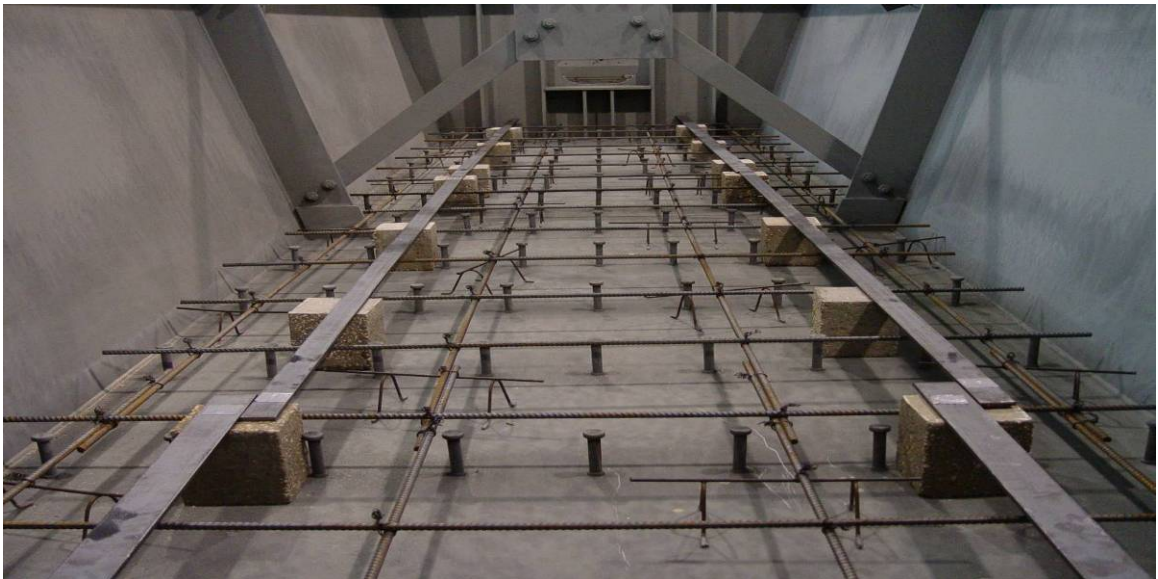
Figure 5.5 Placement of Bottom Concrete Slab
