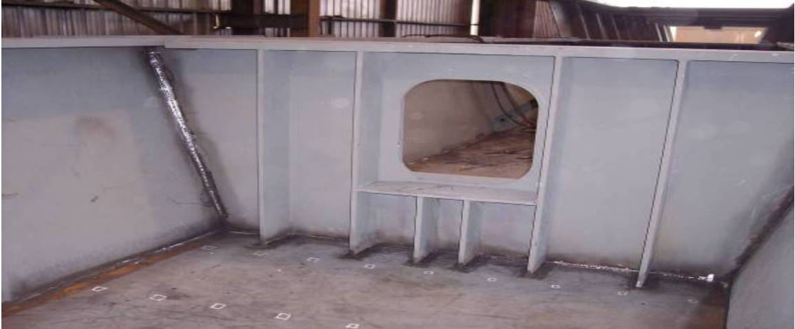
Figure 3.9 Diaphragm Welded to Steel Box
