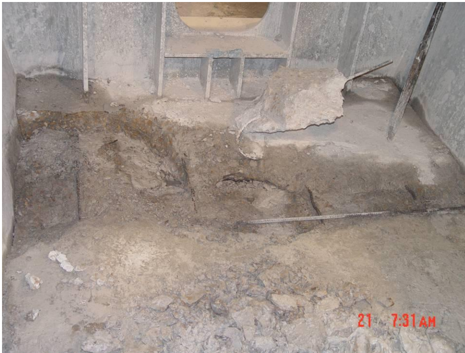
Figure 7: Concrete Failure (Removal of Loose Pieces)
