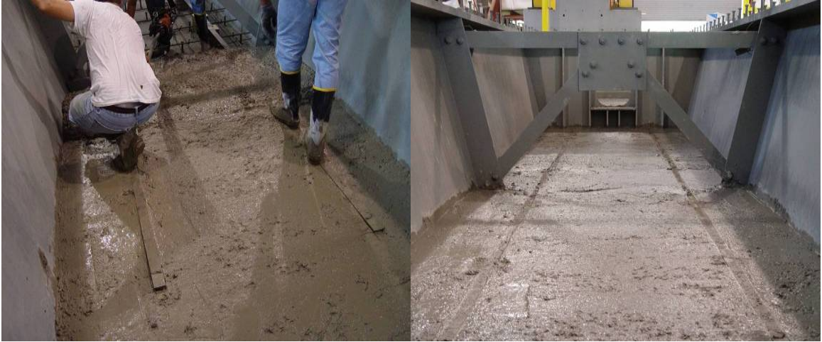
Figure 3.15 Pouring of Bottom Concrete Slab
