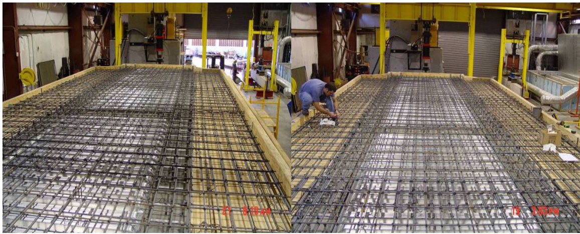
Figure 3.17 Reinforcement for Top Concrete Slab
