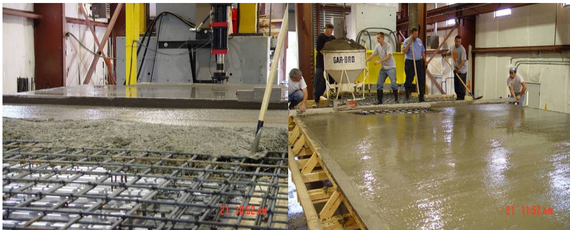
Figure 3.18 Pouring of Top Concrete Slab
