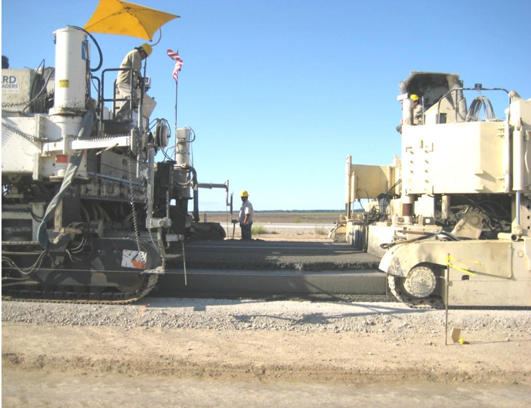
Figure 73: Kansas I-70 two-lift paving operation.
