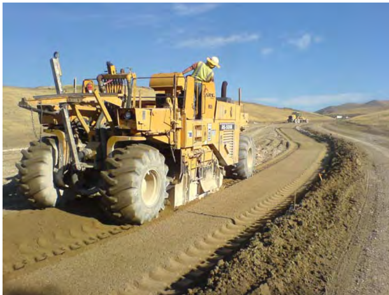
Figure 3-1. Final field mixing of lime-treated soil 1
