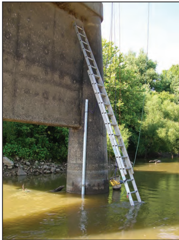
Installation of 3-inch galvanized steel pipe encasing the transducer head and shielded cable on the downstream side of the upstream conical column of pier 4.
