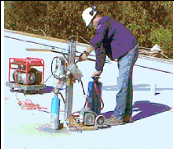
Figure D-1 – Advancing core bit through deck
