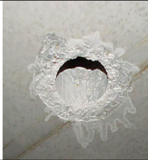
Figure D-2 – Core location as seen from underneath
