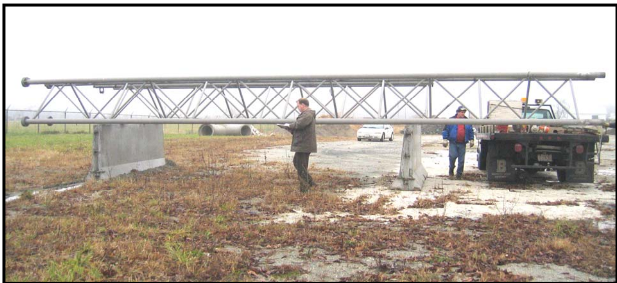
Figure 5: Remnants of Sign Truss at the District 7 Dixie Outpost
