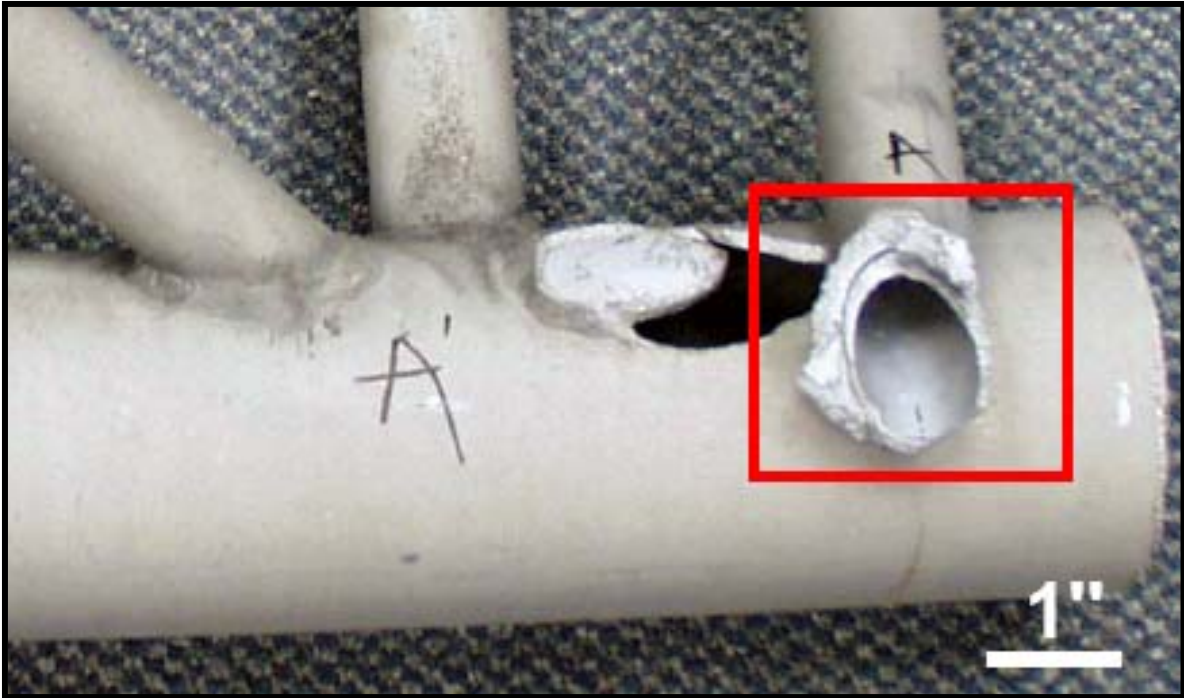
Figure 18: Metallurgical Sample Taken From Upper Chord of Failed Truss
