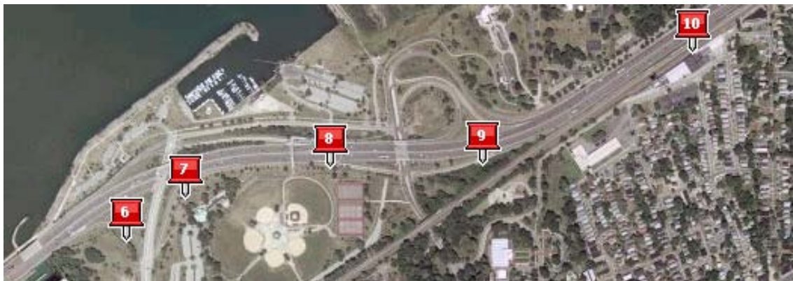
Figure 27. Trailer Locations on I-90 Eastbound after Construction
