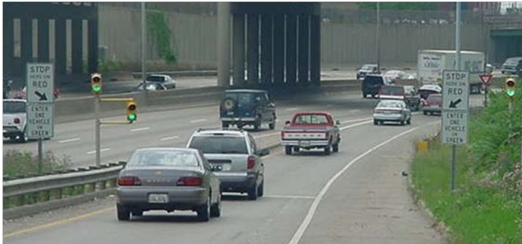
Figure 39. Sample ramp metering signal application at an entrance ramp (from [18]).
