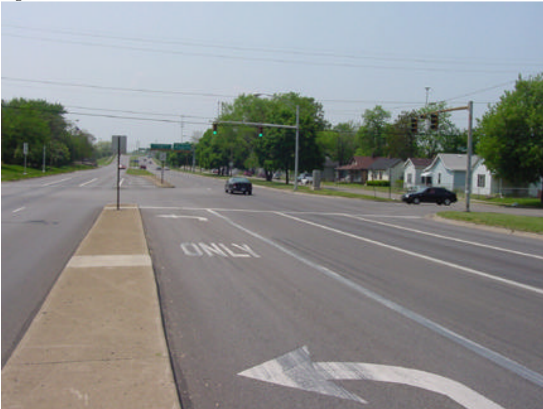
Figure 4. Roosevelt Blvd at Wicoff – Westbound
