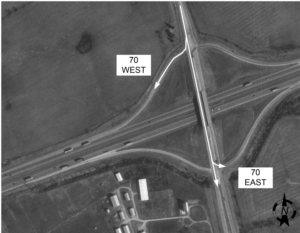
Figure 26. Aerial View of the Plain City Georgesville Road (Southbound) Interchange Site with I 70
