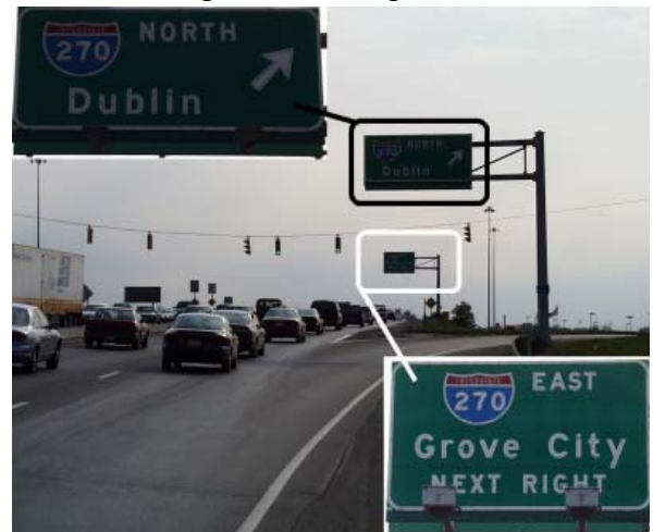
d. Cantilever Overhead Signs Before and at First Gore
