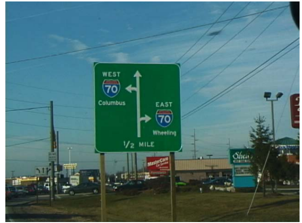
b. Shoulder Mounted Diagrammatic Sign 1/2 Mile Ahead of Gore, Located just ahead of Chantry Rd
