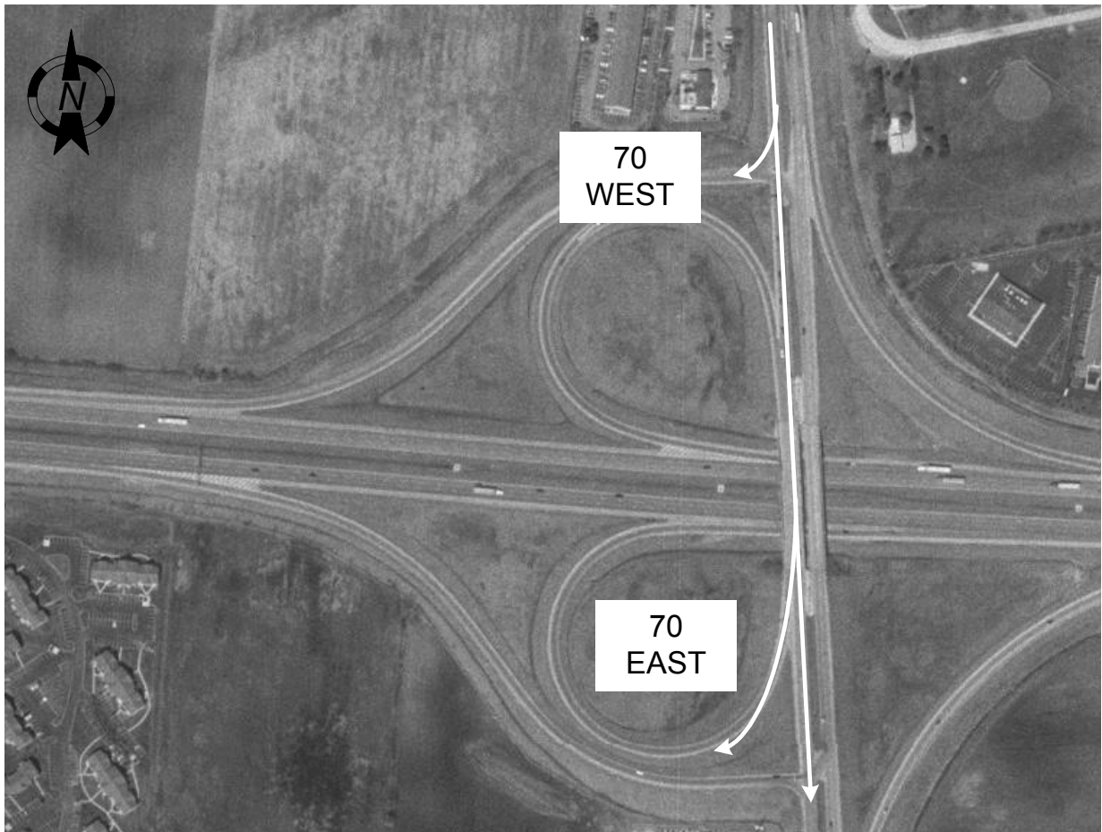
Figure 22. Aerial View of the Hilliard Rome Road (Southbound) Interchange Site with I 70
