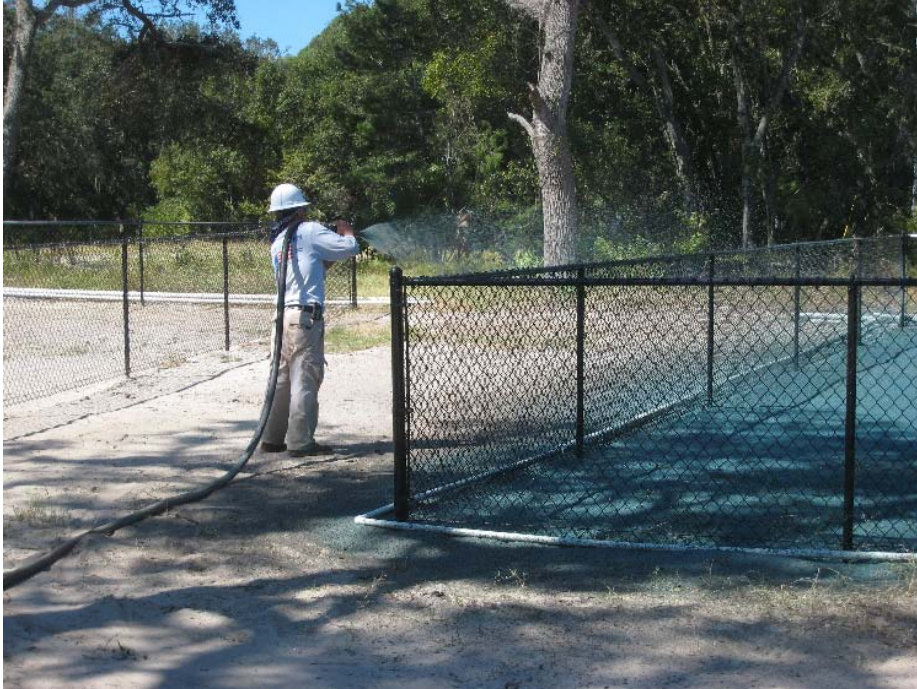
Figure 8. Hydroseeding common bermudagrass.
