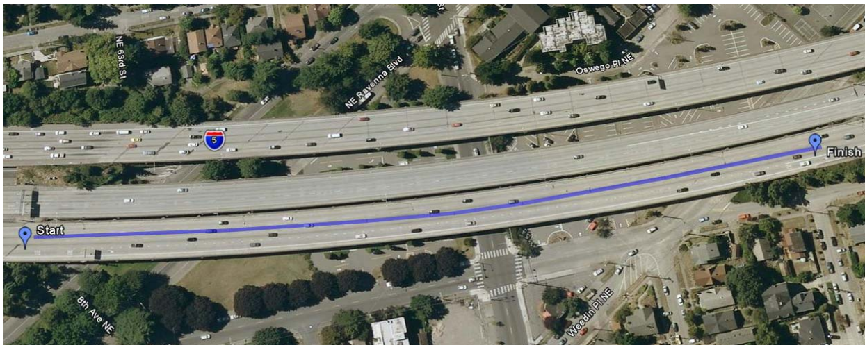
Figure 4.1. Aerial view of the I-5 Ravenna Bridge
