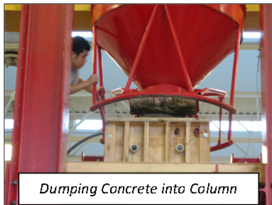
Figure 3.18 Concrete Pour for Foundation and Column
