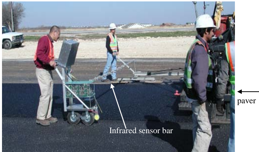
(a) Infrared sensor bar behind paver screed
