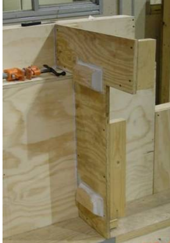
Figure 31 – Form for shear keys
