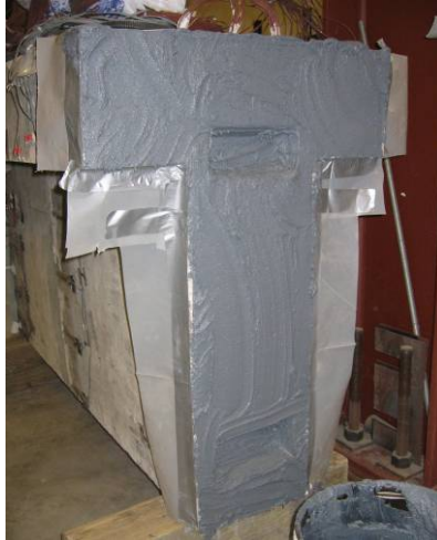
Figure 229: Epoxy applied to match-cast face at joint
