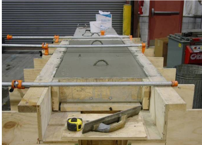
Figure 34 – Match-casting of segment
