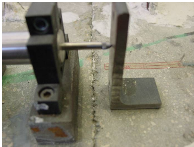
Figure 109 – Condition of joint J2 on top of flange
