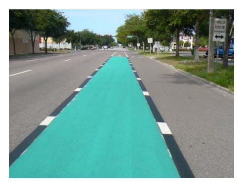
Figure 4. Black mini-stripes added to border of green bike lane weaving area.
