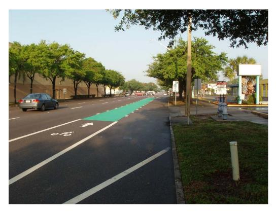
Figure 2. First "after" condition for green bike lane weaving area.
