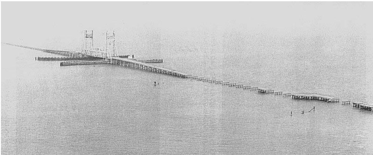
Figure 1- 1 Damage to Dauphin Island Causeway (Alabama) caused by Hurricane Frederic.
