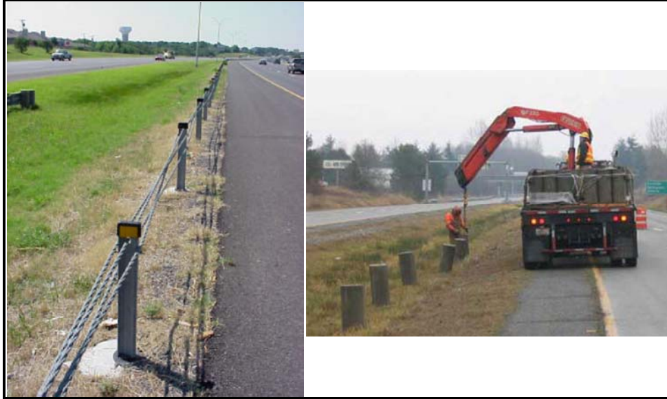
Figure 3-1. Posts in Concrete Drilled Shafts with Sockets.
