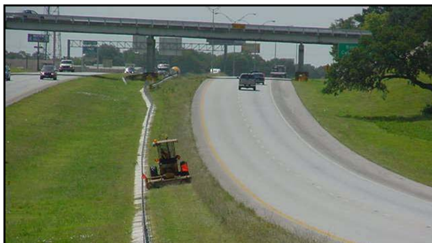
Figure 2-34. Concrete Mow Strip in Texas.
