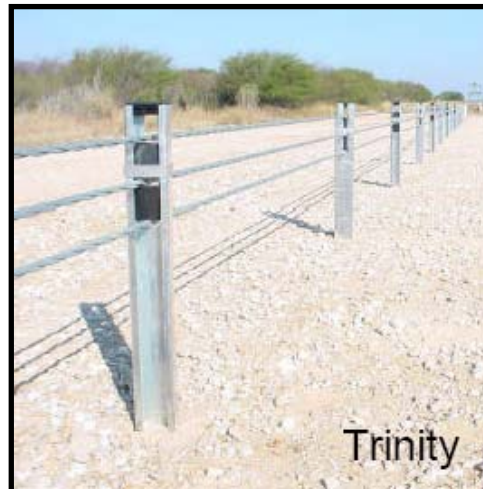
Figure 2-9. Trinity CASS Barrier.
