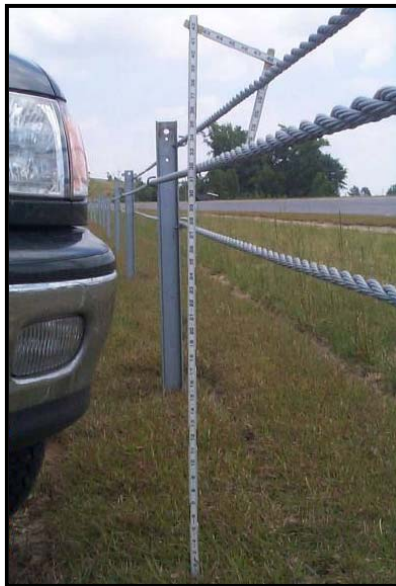
Figure 2-15. Cable Height.
