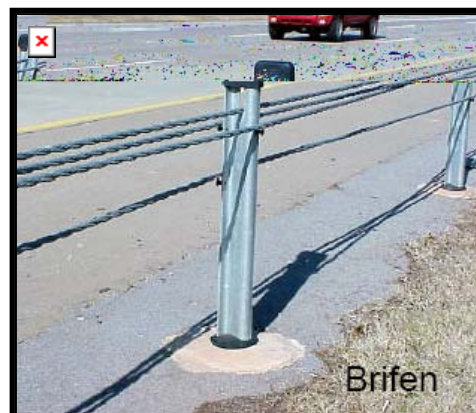
Figure 2-6. Brifen Wire Rope Safety Fence.
