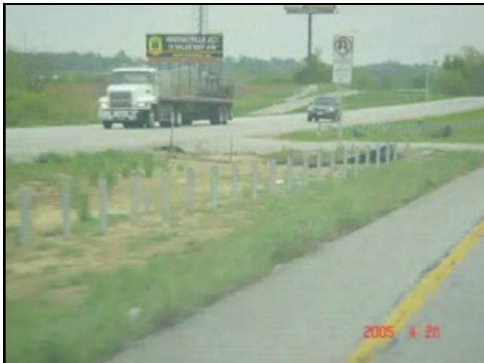
Figure 2-39. Picture Showing a Typical Emergency Crossover.
