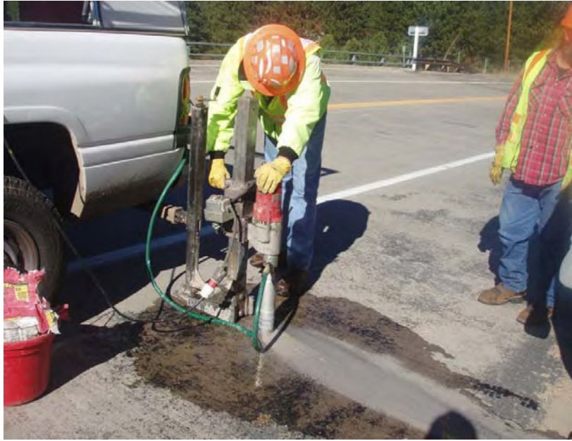
Figure 7. Bridge deck coring
