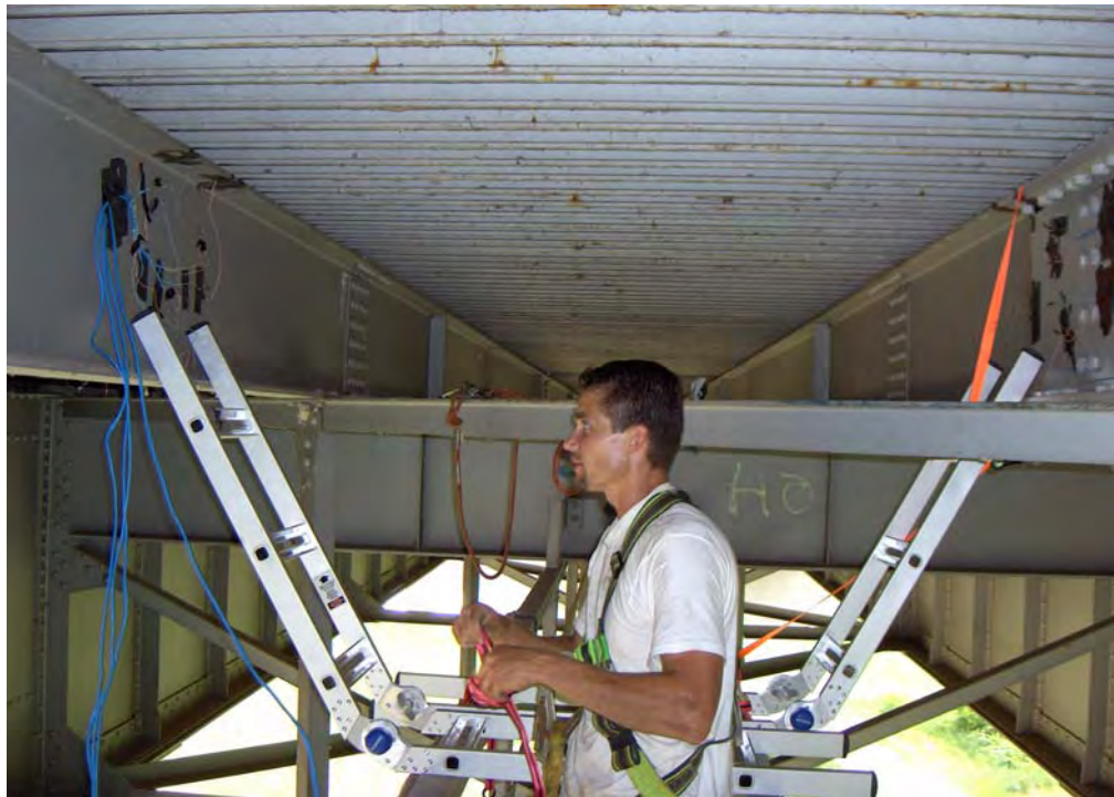
Figure 7-4. Strain gage installation.
