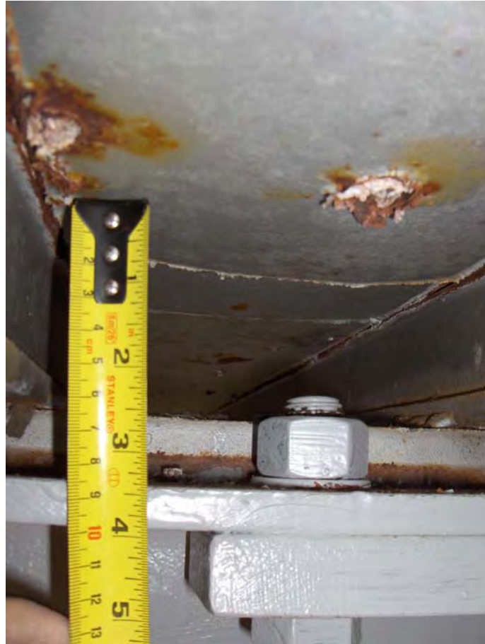
Figure 9-1. Limited space available for work on joints.
