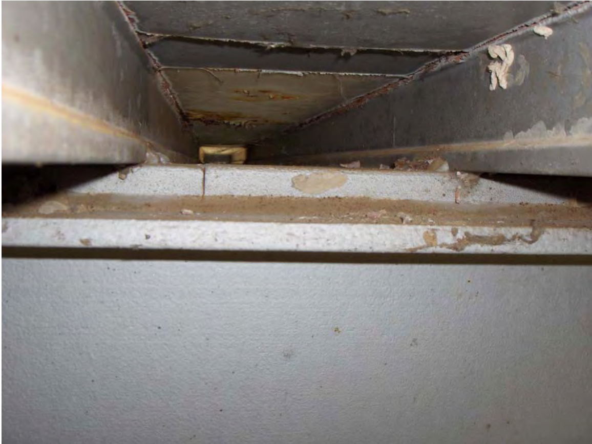
Figure 3-5. Similar butt joint weld detail located near cracked stringer on east approach.
