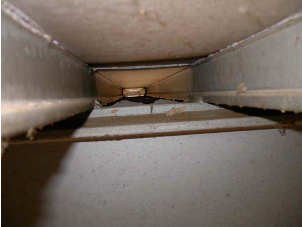
Figure 2-8. Transverse view of grid deck welded to shim plate on top flange of stringer in plate girder spans.
