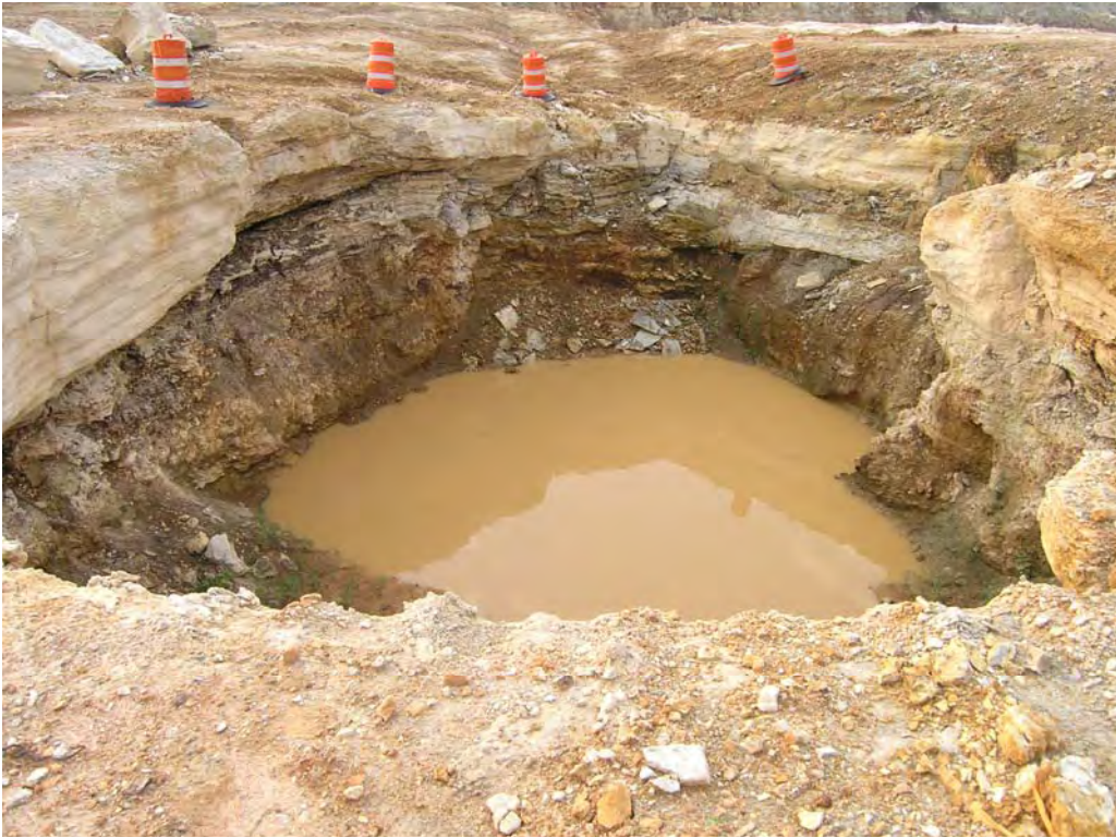
Figure 12: Photograph of the sinkhole, taken from a location immediately to the south of the feature.
