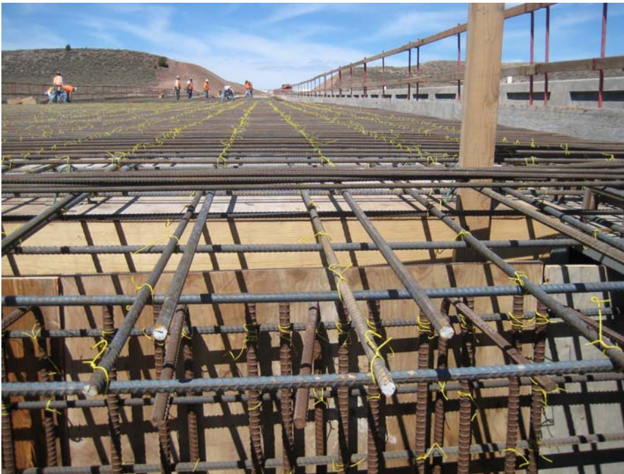
Figure 5.4. Abutment MMFX Deck Steel
