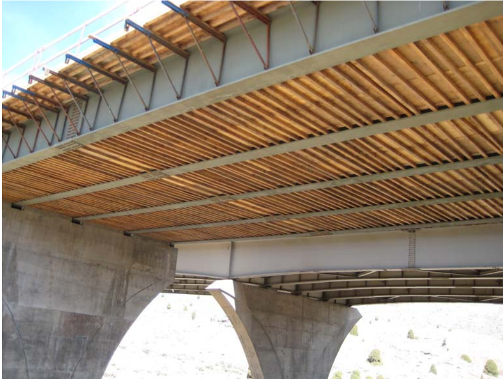
Figure 5.2. Steel Girders of MMFX Deck Bridge
