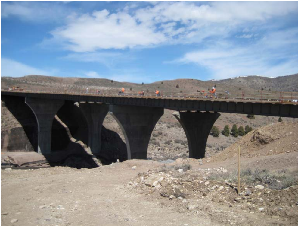
Figure 5.1 Elevation View of MMFX Bridge.
