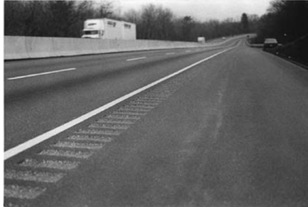
Figure 4: Sonic Nap Alert Pattern (SNAP) Rumble Strip
