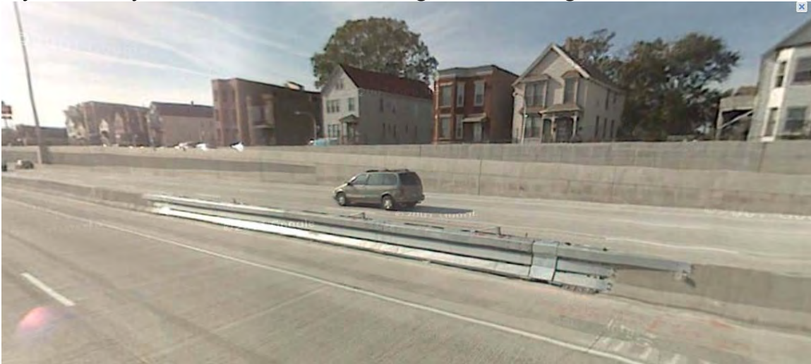
Figure 6 Example of a temporary barrier gate for express lane emergency access (by Barrier Systems) in barrier wall along I-94 in Chicago, IL
